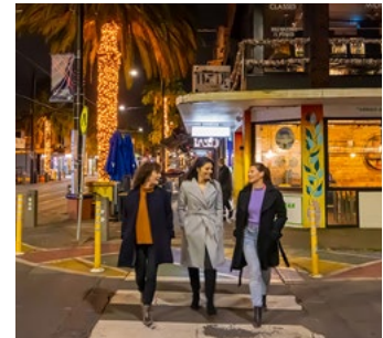
New creative lighting was installed along Acland Street, adding vibrancy to the area.
