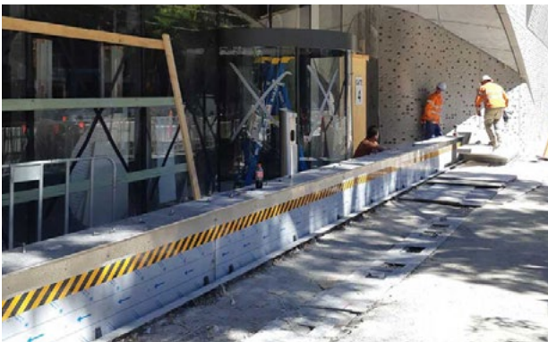
Figure 72: The barrier is concealed beneath the pavement with a top plate, side panels and drainage system integrated into the paving.
