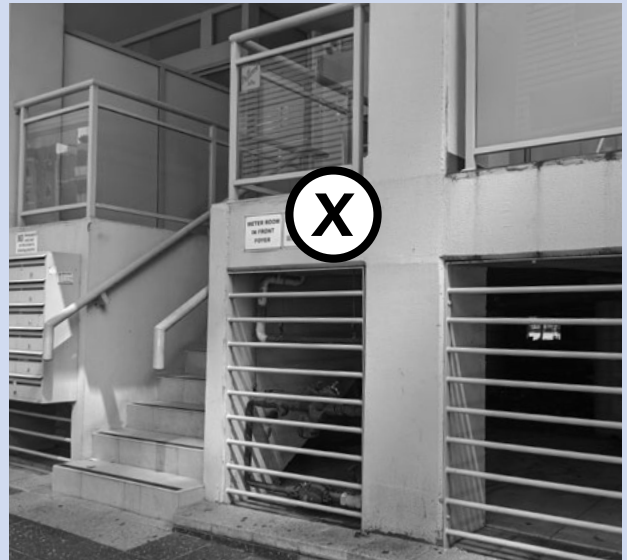
Figure 60: The interface must be carefully designed to ensure a positive relationship to the street. This example shows a raised ground floor to allow for water to flow underneath the building. It has resulted in a dark enclosed space at street level that regularly gets filled with rubbish.
