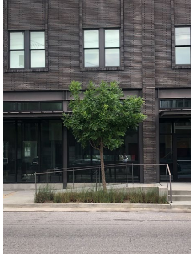
Figure 15: Raised footpath along a section of the street allows for accessible transition between two levels.
