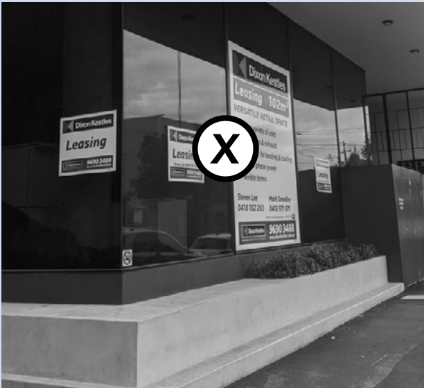
Figure 59: While a concrete plinth has a potential to offer seating, it does not create an inviting space to sit when combined with a large expanse of dark glazing.
