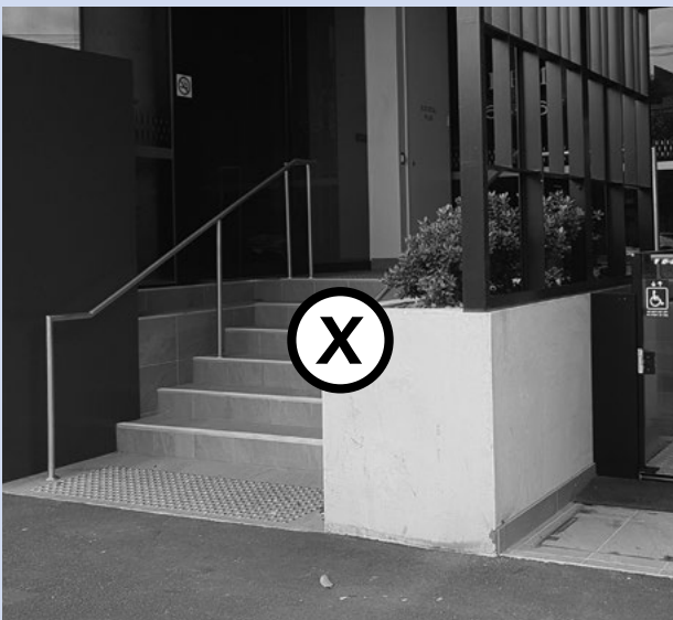
Figure 34: The presentation and legibility of the main entry to the building is compromised because it is recessed from the street. An external platform lift is not a preferred outcome
