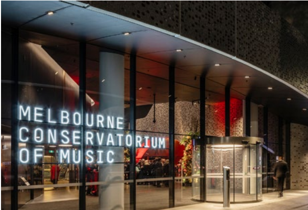
Figure 71: The welcoming public entrance to the Ian Potter Southbank Centre has well concealed flood protection in the form a self-actuating barrier that rises vertically 1 metre in response to incoming flood waters.
