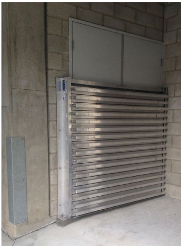
Figure 62: A retrofit example of manually installed segmented flood barriers to protect building services during flood events.
