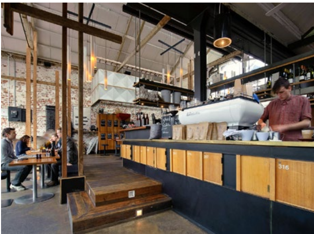
Figure 66: Polished concrete floors, brick walls and hardwood timbers provide resilient finishes.
