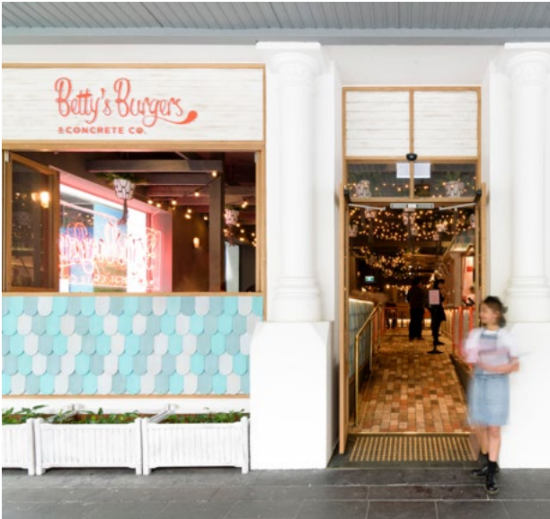
Figure 47: An internal ramp inside this cafe's main entrance provides universal access up to the elevated internal floor level. Large bi-fold windows above flood level provide a good visual connection to the street.
