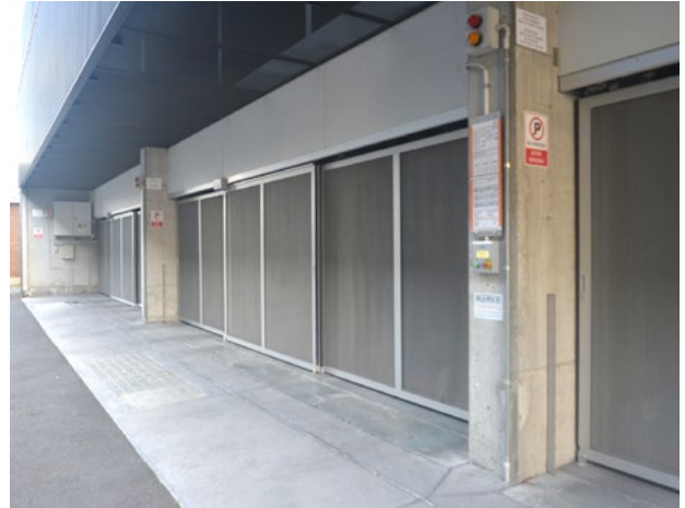
Figure 69: Self-actuating vertical-rise flood barriers protect these garages with car stackers in a South Melbourne laneway.
