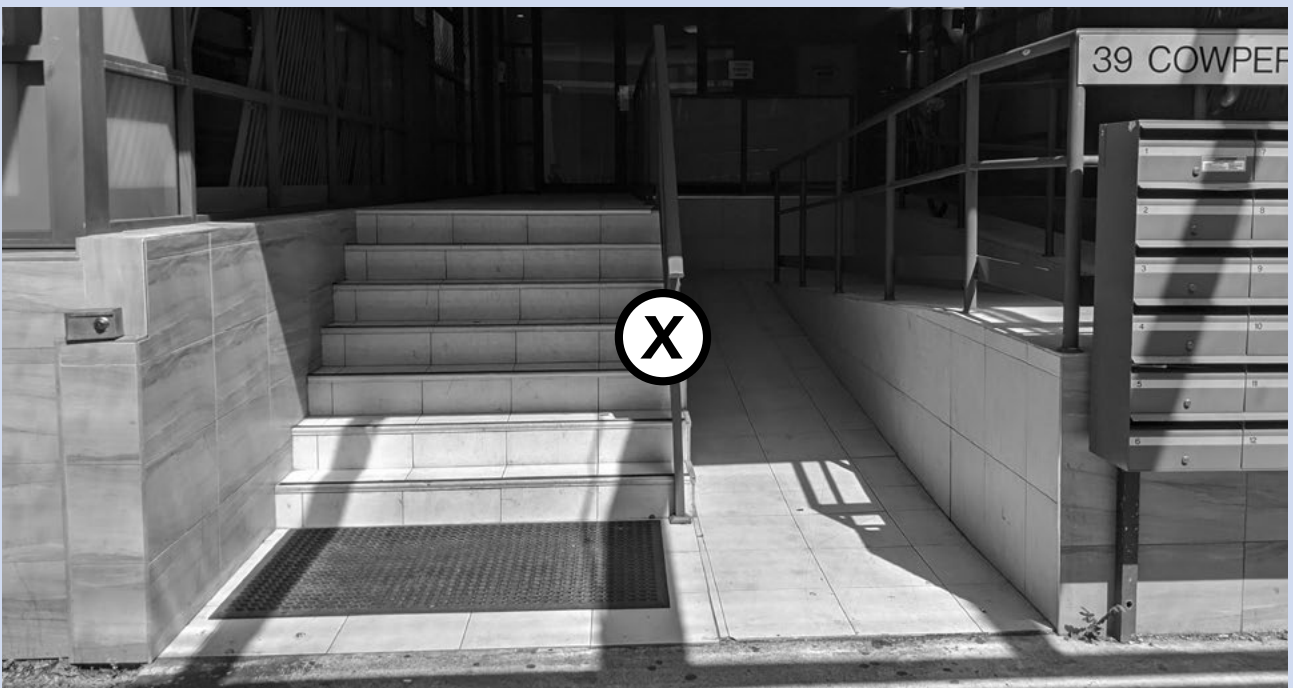
Figure 45: A long ramp into the building can create a dark entrapment space.
