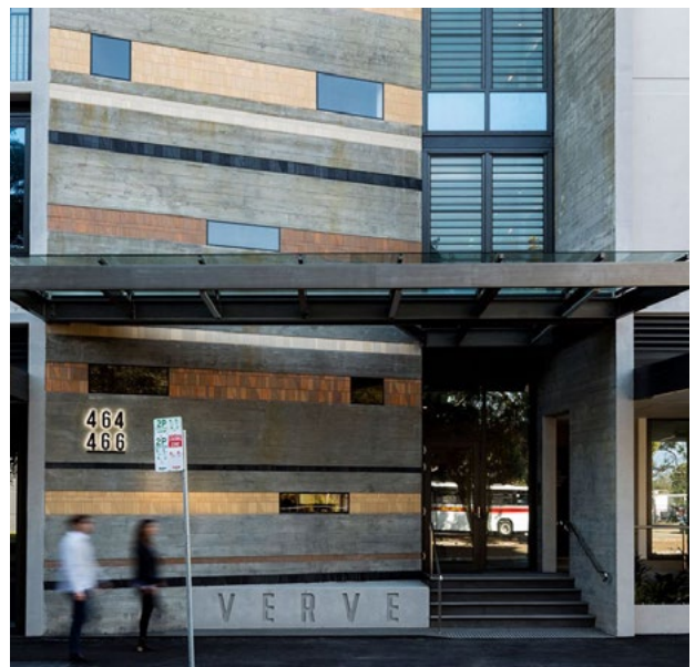
Figure 65: Concrete plinth with integrated building signage and a raised planter bed provide a flood resilient base to the elevated entrance to this apartment building.
