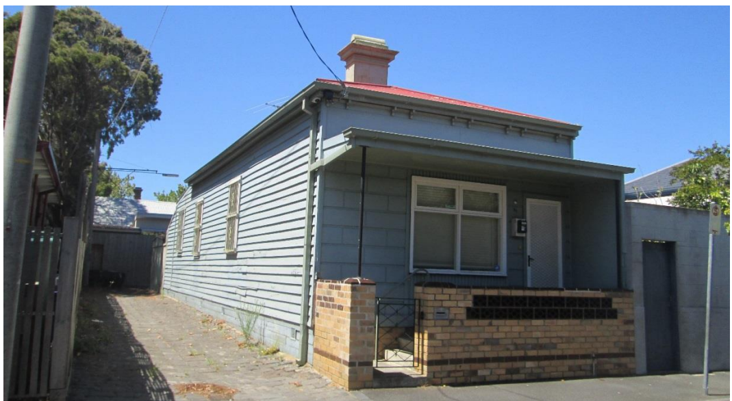
Figure 3. Photographs of the front façade of the existing dwelling at No. 61 Neville St.
