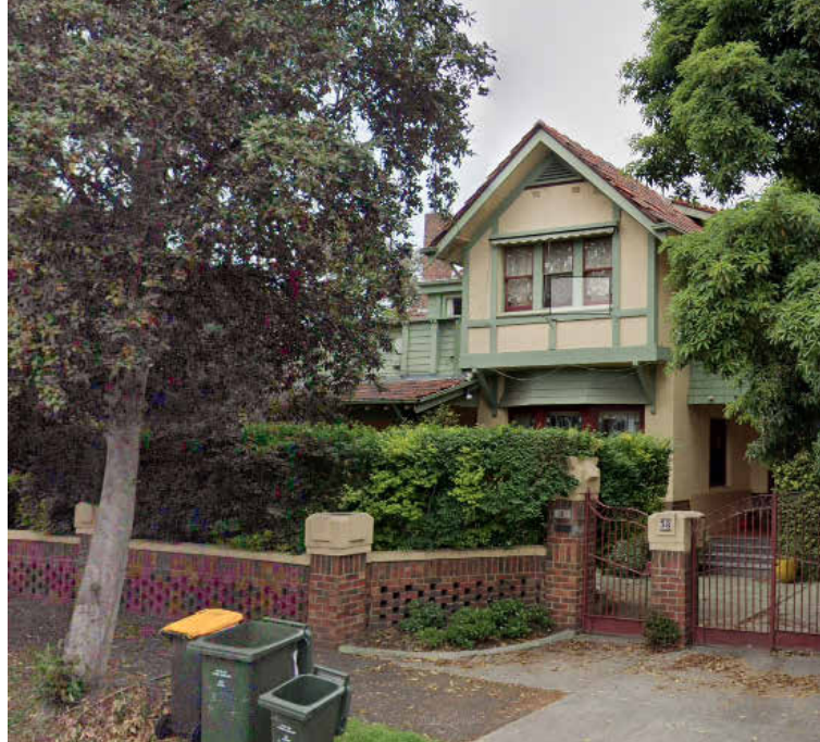
38 EILDON ROAD - RESIDENTIAL PROPERTY
