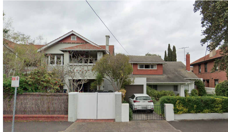
34 EILDON ROAD - RESIDENTIAL PROPERTY
