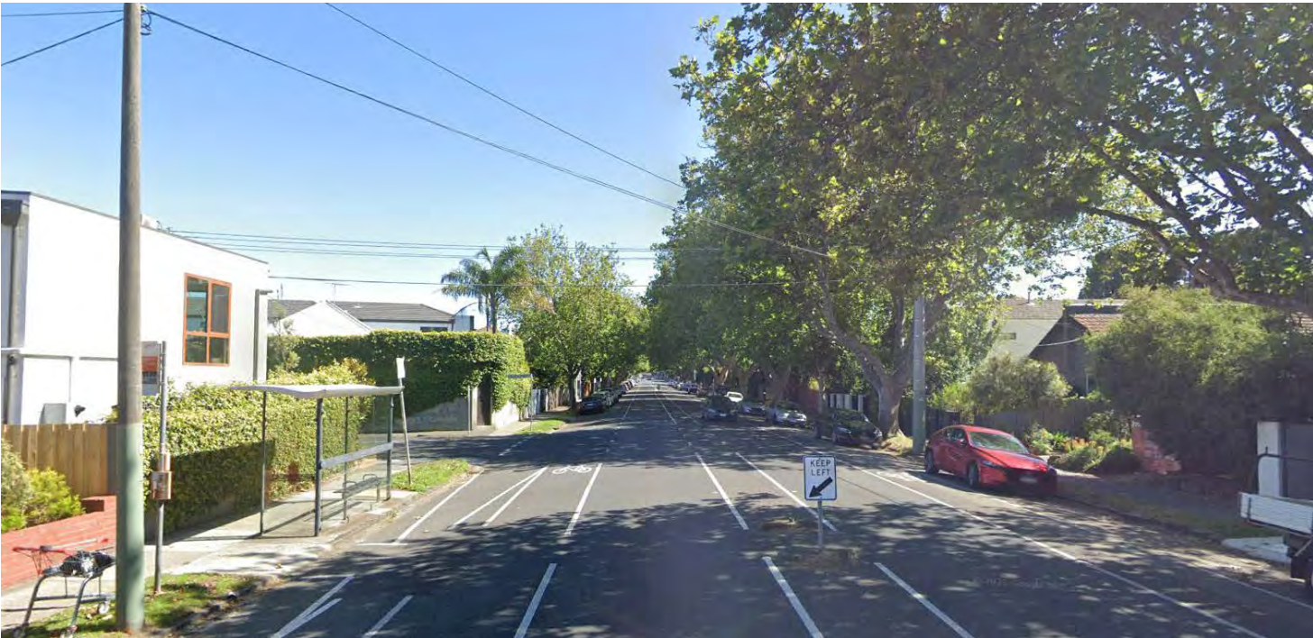
Figure 30: Barkly Street in St Kilda is an example of a Movement Street
