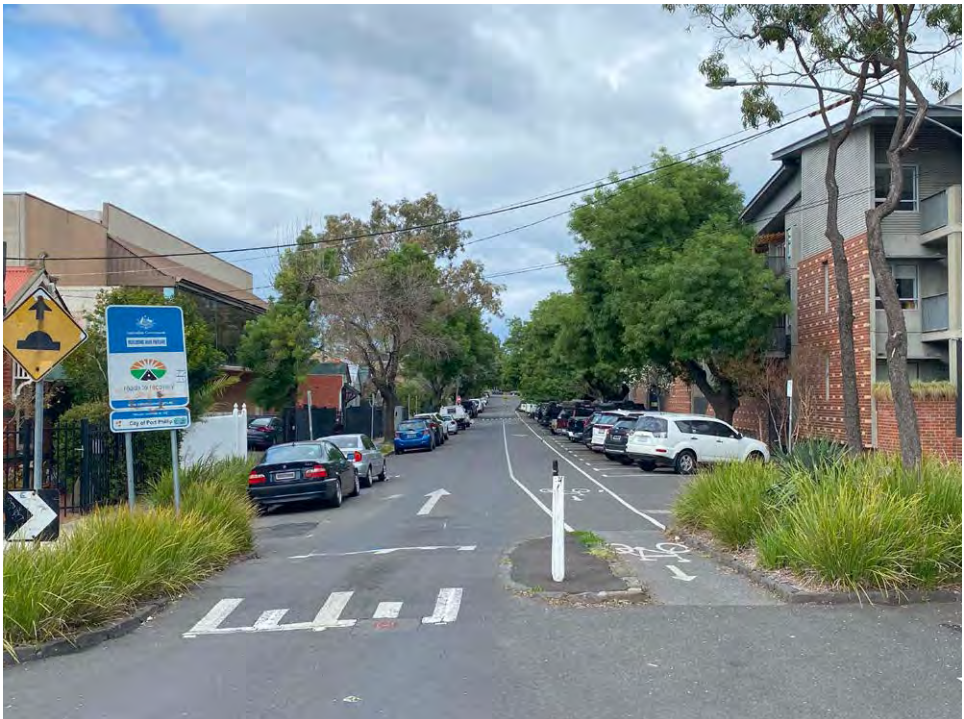
Figure 36: Combined one way street and bike lane along Greeves Street
