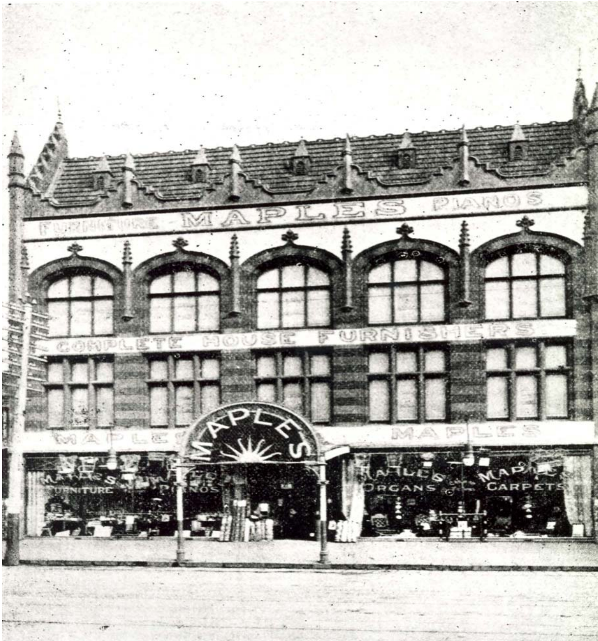
Maples Furniture Warehouse, 1905 258–264 Clarendon Street
