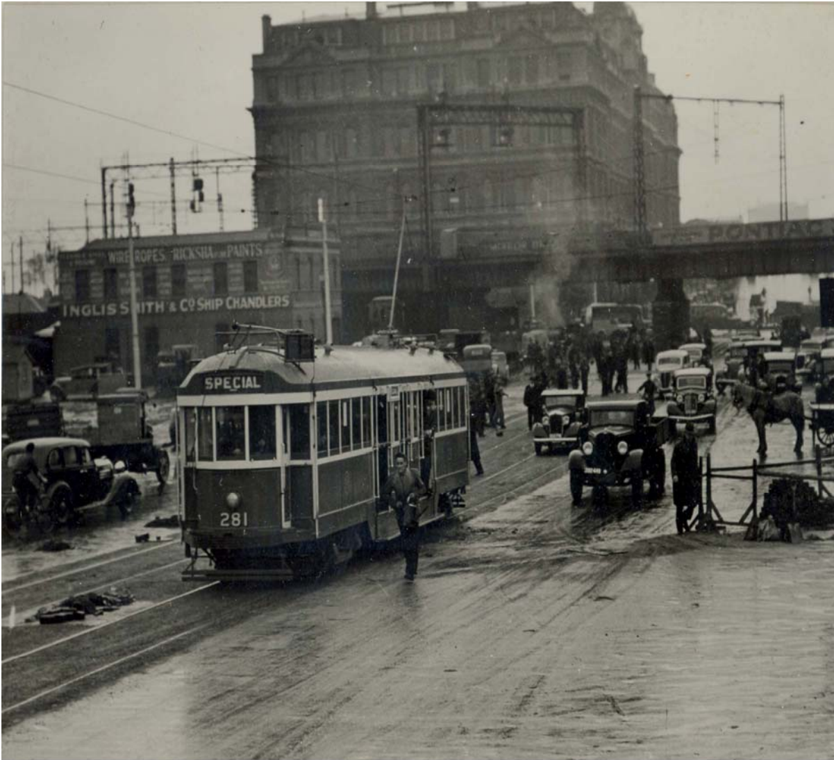
Ceremony, driving of the first tram on the new South Melbourne Electric Tramway, Clarendon Street, Saturday 24 July 1936.
