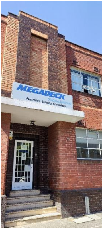
View of the recessed front entrance. Note the projecting brickwork pattern.
