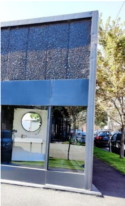
View of the corner at Coventry Street and Eastern Road showing the original entrance location. Note also the textured pre-cast concrete panels in vertical divisions, and the continuous form of the column to the parapet edge.
