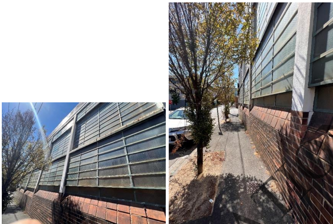
Detail views of the glazing and clinker brick base. Note the glazing steps in and out to provide gaps for ventilation.
