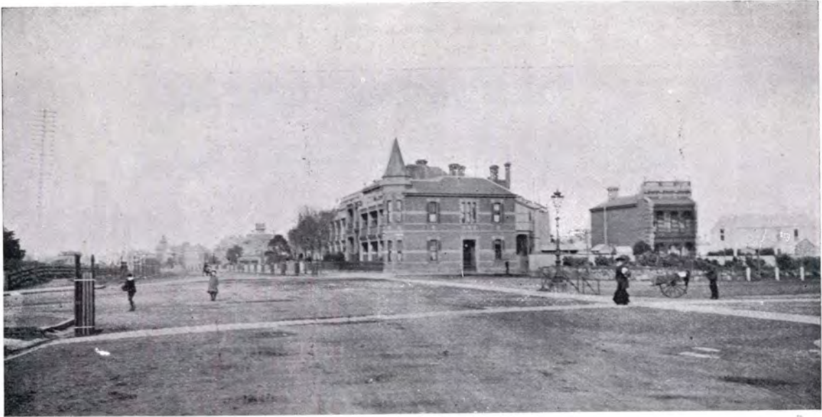
Canterbury Road from Kerford Road.
