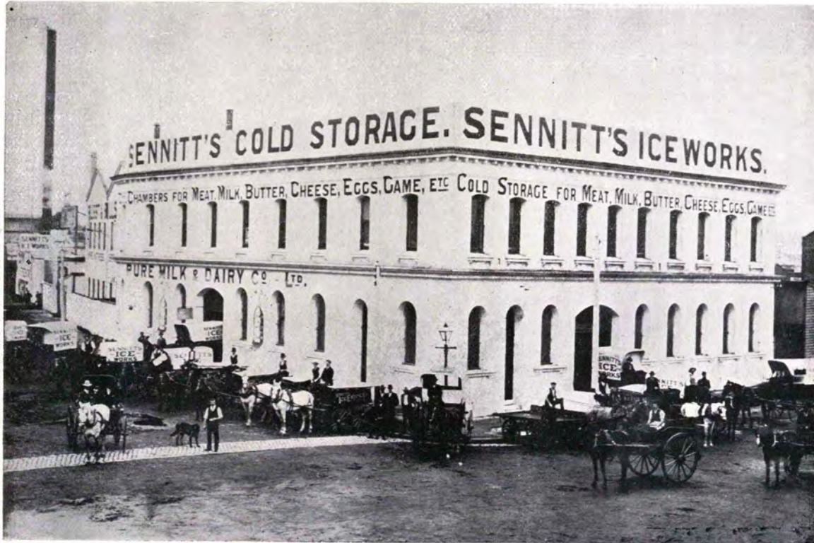
Sennitt's Cold Storage & Ice Works, Yarra Bank,
