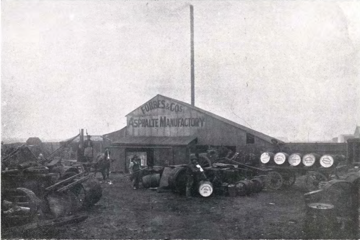
View of Forbes & Co's Asphalte Factory.
