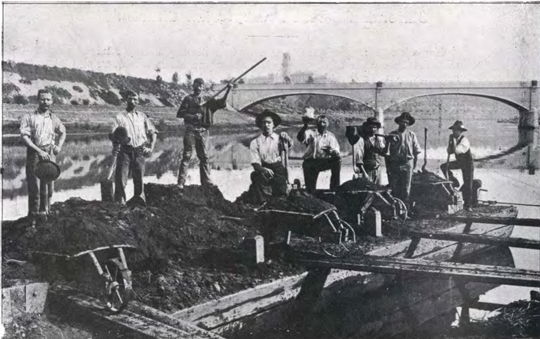
River Improvements since the Great Flood.
