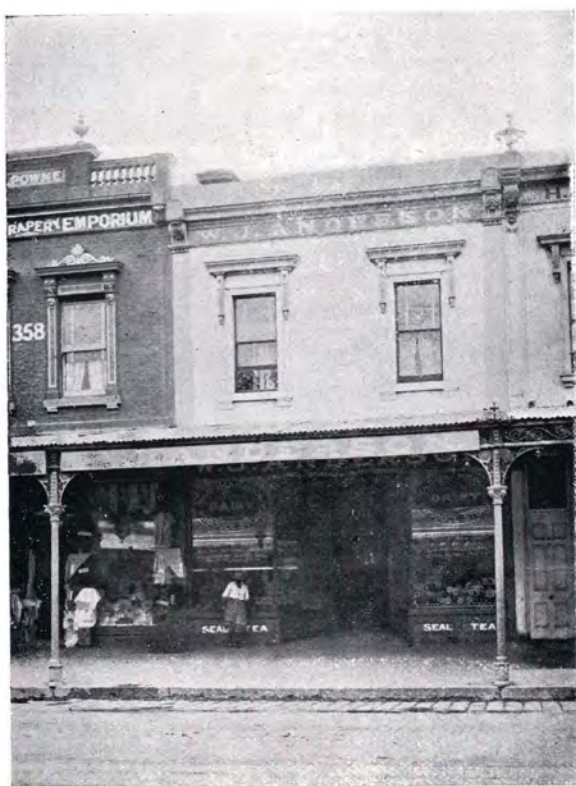
Anderson's Dairy Produce Store, 356 Clarendon St.
