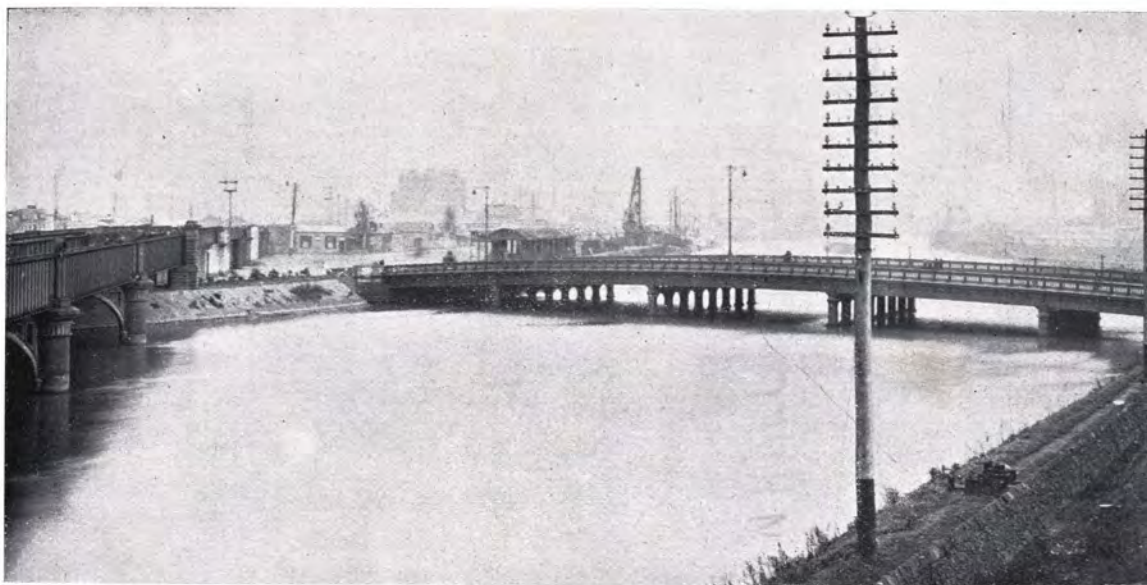
Queen's Bridge and Railway Bridge.
