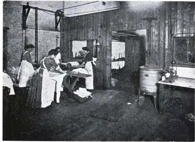
Corner of Starch Room, Albert Park Steam Laundry.
