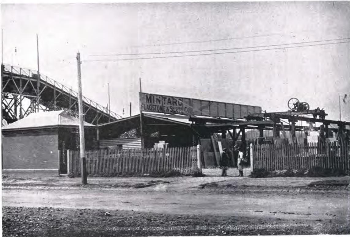
Mintaro Slate Works, Sturt Street.
