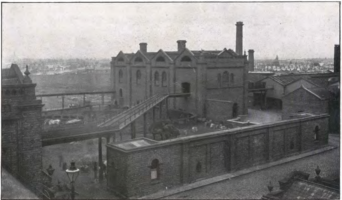
View of Retort House and Coke Yards, South Melbourne.
