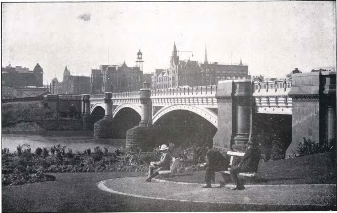
Princes Bridge, from South Melbourne Side.
