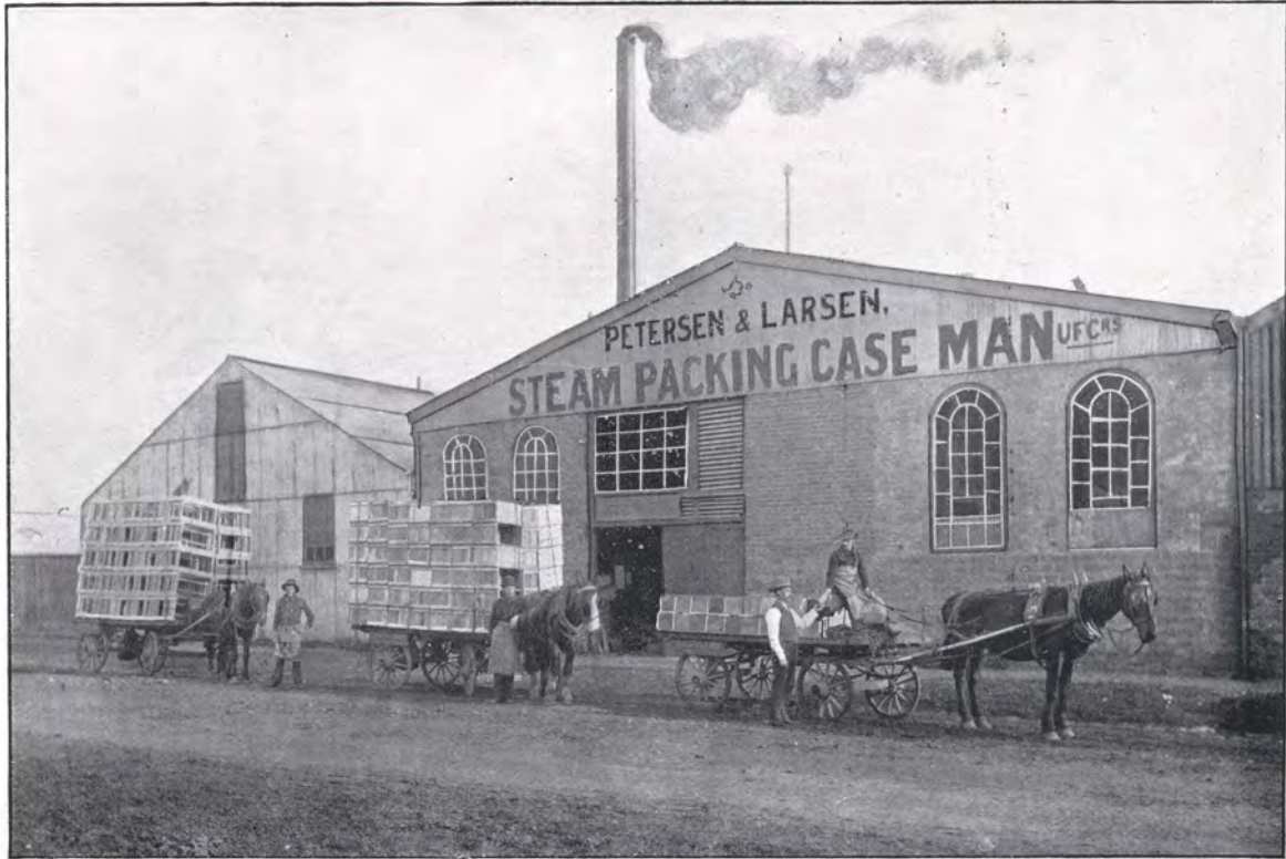
Petersen & Larsen's Offices & Box Factory, Normanby Rd.
