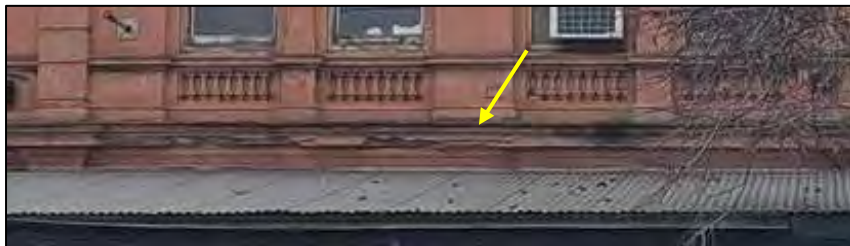
Figure 23 Detail view of the damaged render to string course.
