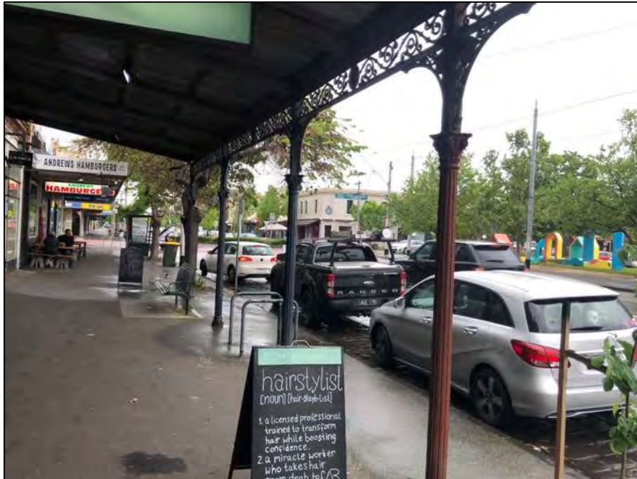
Figure 8 A verandah supported by cast iron posts extends across the facade of 148 & 150 Bridport Street.
