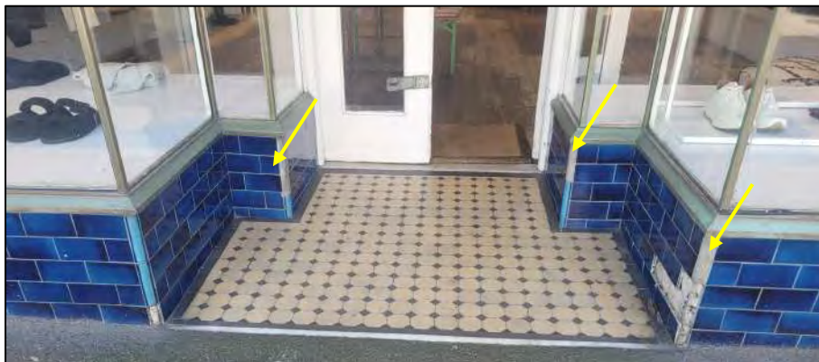
Figure 17 Detail view of the tiles to shopfront plinth and the shop ingo floor to be retained and restored.
