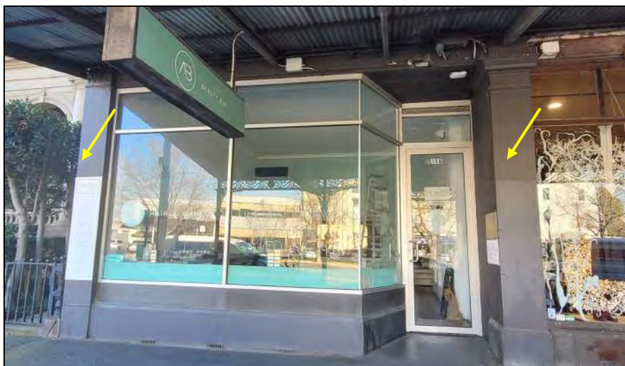
Figure 22 View of the granite pillars including mouldings to either side of shop 150 to be retained and restored.
