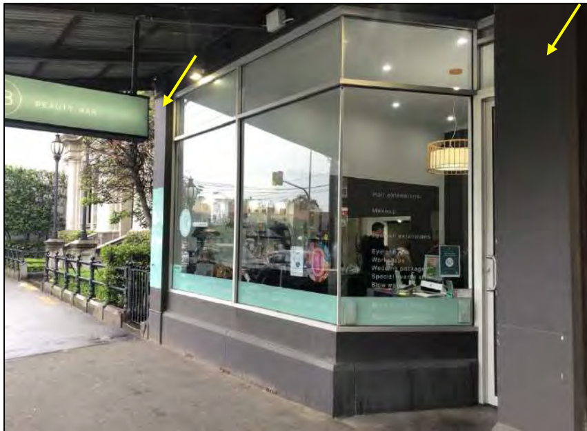
Figure 12 Existing shopfront to number 150. Granite to the pillar's to be retained, shop front to be demolished.
