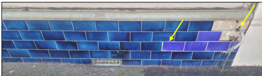
Figure 18 Detail view of the tiles to the shop plinth to be retained and restored including replacement of the non-matching tiles.
