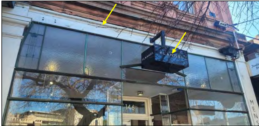
Figure 19 Detail view of the metal verandah bracket to be retained and non-original sign to be demolished.
