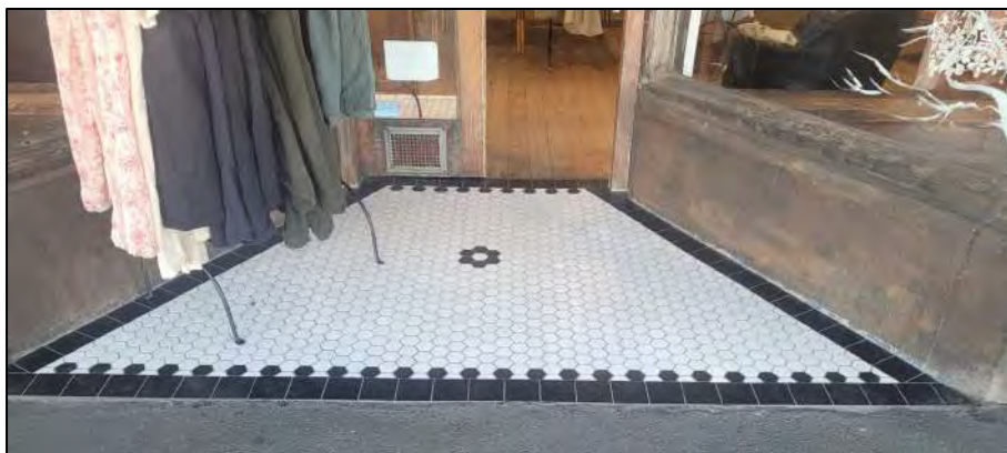
Figure 20 Detail view of the tiles to shop ingo floor to be retained and restored.
