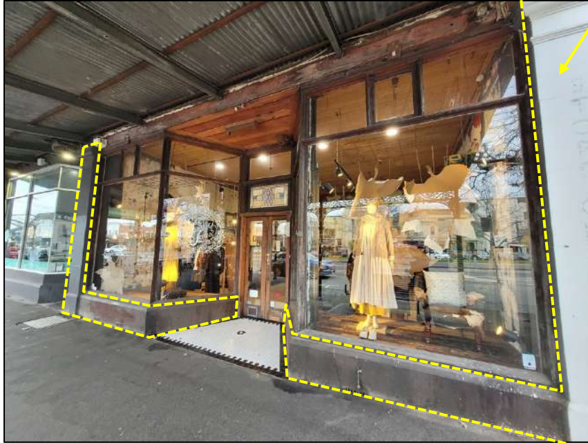
Figure 13 Existing shopfront to number 149 with the granite overpainted. Paint is to be removed and the granite restored.
