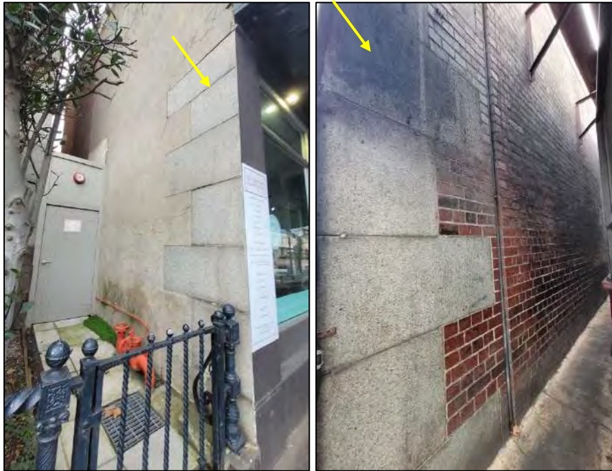
Figure 15 The existing granite to both side elevations, to be cleaned and mortar renewed.
