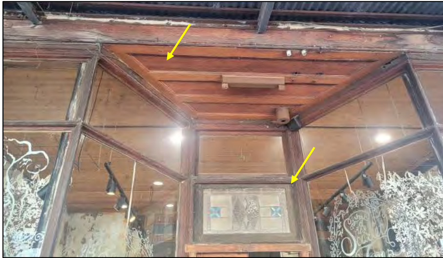
Figure 21 Detail view of the tiles to the shop ingo ceiling and leadlight windows to be retained and restored.
