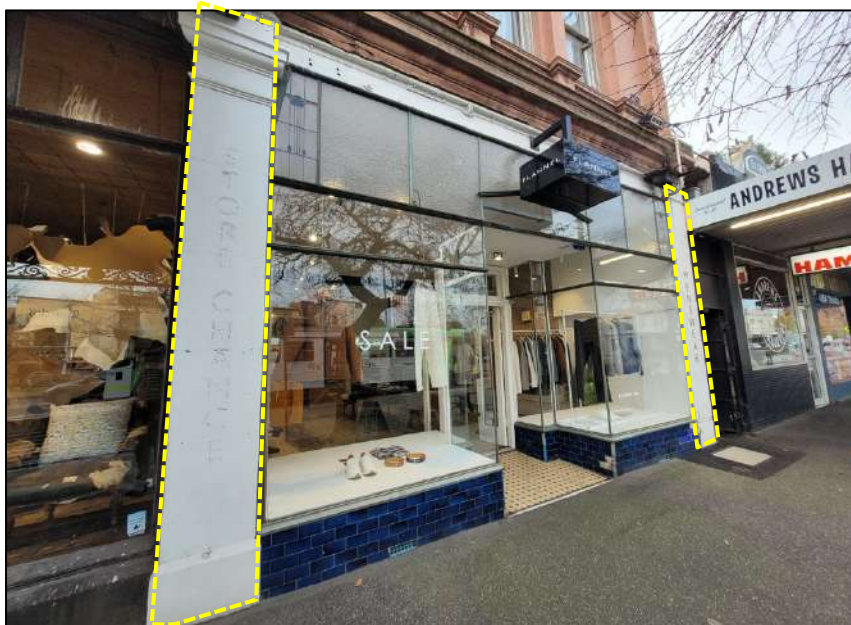
Figure 14 Existing granite pillars to number 146 that have been overpainted. Paint is to be removed and the granite restored.
