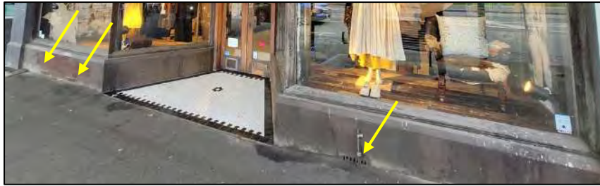
Figure 11 Half buried air vents.
