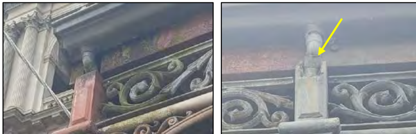
Figure 27 Detail of the downpipes inserted into the verandah column; note the damage to column in the image to the right.
