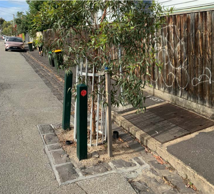
An example of a tree outstand with a flush bluestone kerb, rather than a raised kerb.
