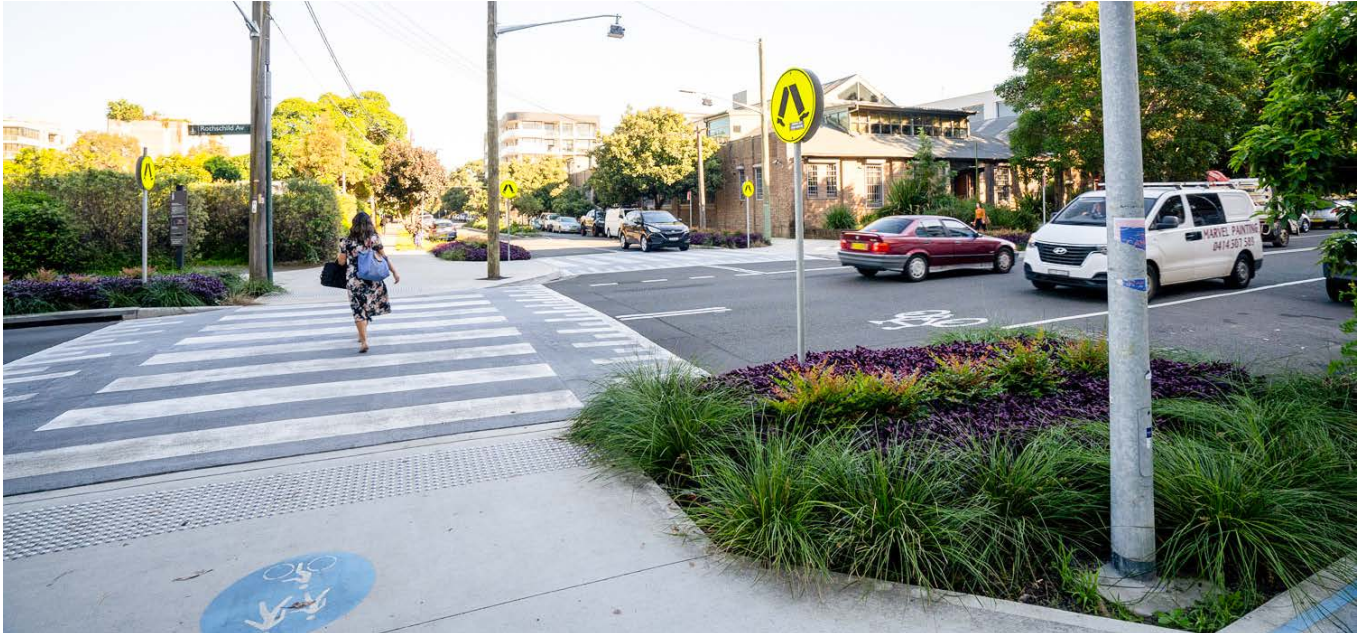
A raised crossing with planting areas created in the adjacent build-outs (Image Credit NSW Government)
