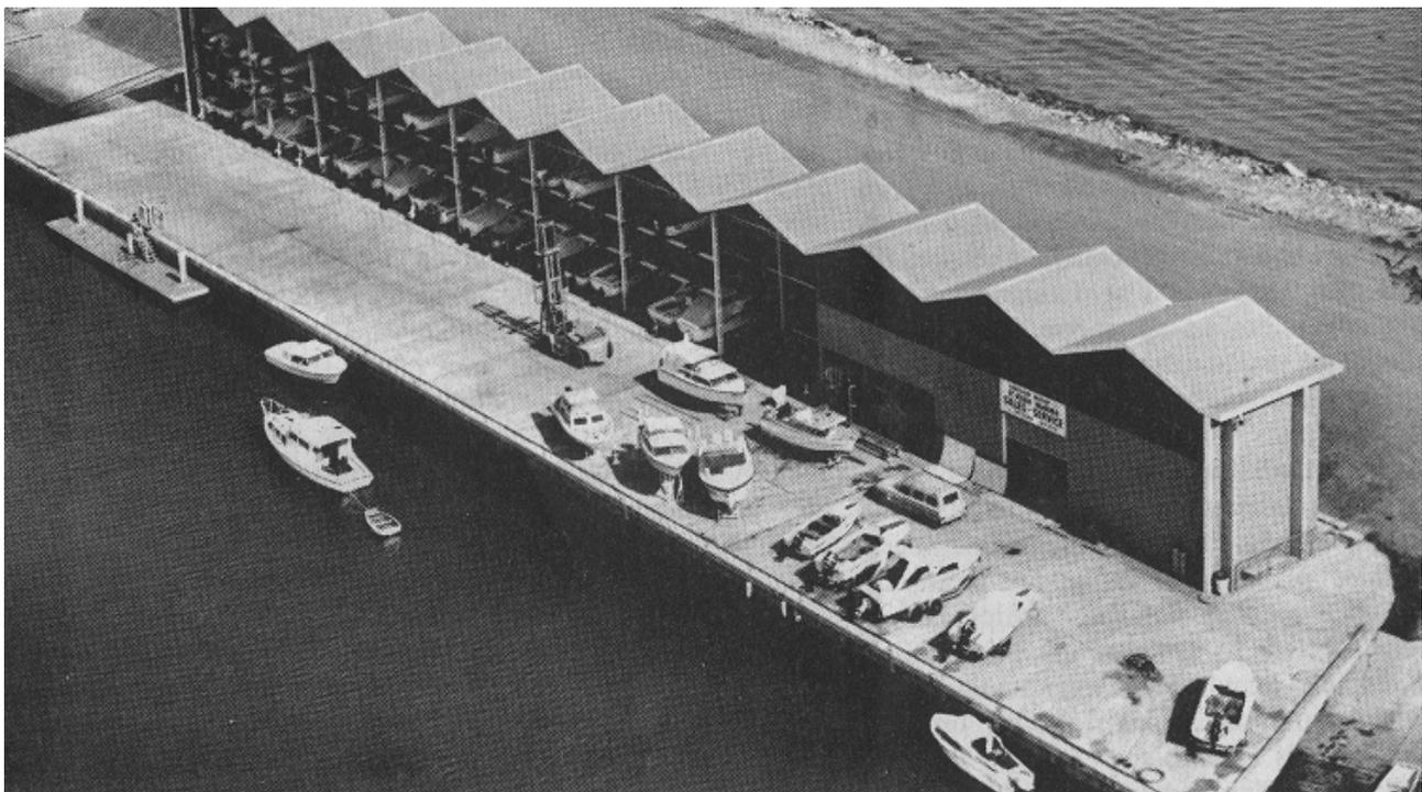
Figure 5: View of the north dry boat storage building in operation (note special forklift truck)
