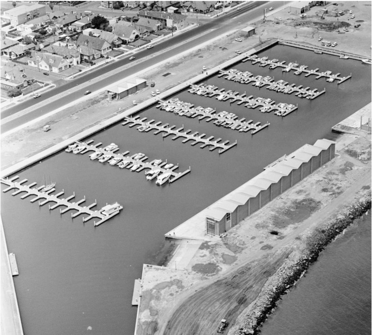
*Figure 3: Marina site circa early 1968, showing moorings, one completed dry boat storage building (with another under construction). Note, on far side of harbour, the amenities block, substation and petrol station. Source: National Archives of Australia (Series A1200, control symbol L79971; photographer uncredited)*
