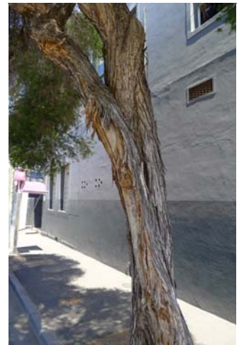
Photo 6 from north-east: Tree 2 vehicle impact damage to stem
