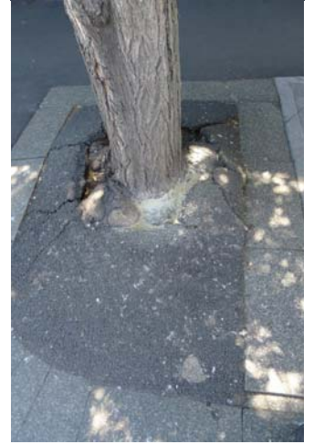
Photo 3 from south: Tree 1 upheaval of hard surfaces around tree
