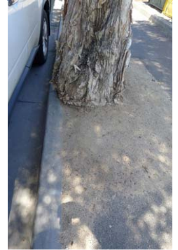
Photo 12 from north: Tree 6 stem has filled out planting space
