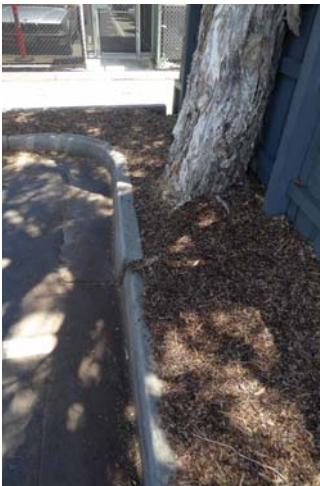
Photo 16 from southeast: Tree 9 kerb has moved due to structural root growth
