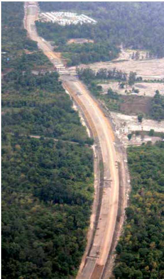
New Suai to Viqueque road under construction.
