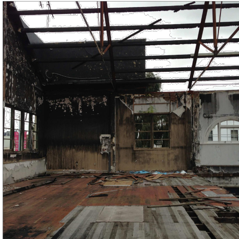
D Interior First Floor - Looking towards Liardet St.
