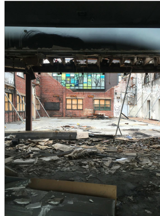
B Interior - Looking towards Kyme Place
