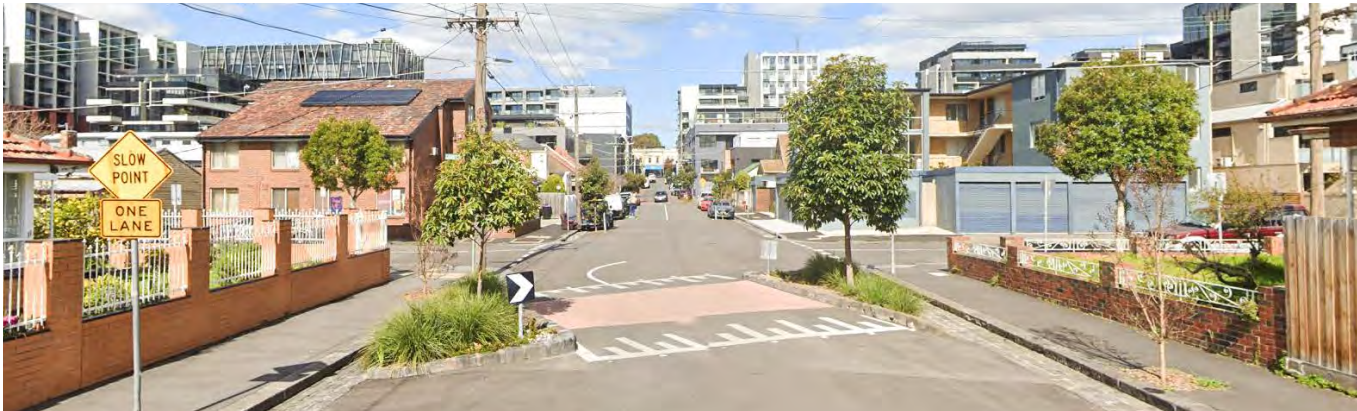
An example of a chicane in Richmond on a typical width street (approximately 15m) that creates space for two trees, understorey planting, and the continuation of two directions of vehicle traffic (Image Credit Google Street View).
