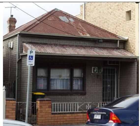
Figure 52. 280 Ross Street. Alterations: removal of front chimney, eaves brackets and verandah, reformatting front window, recladding with fake brick.
