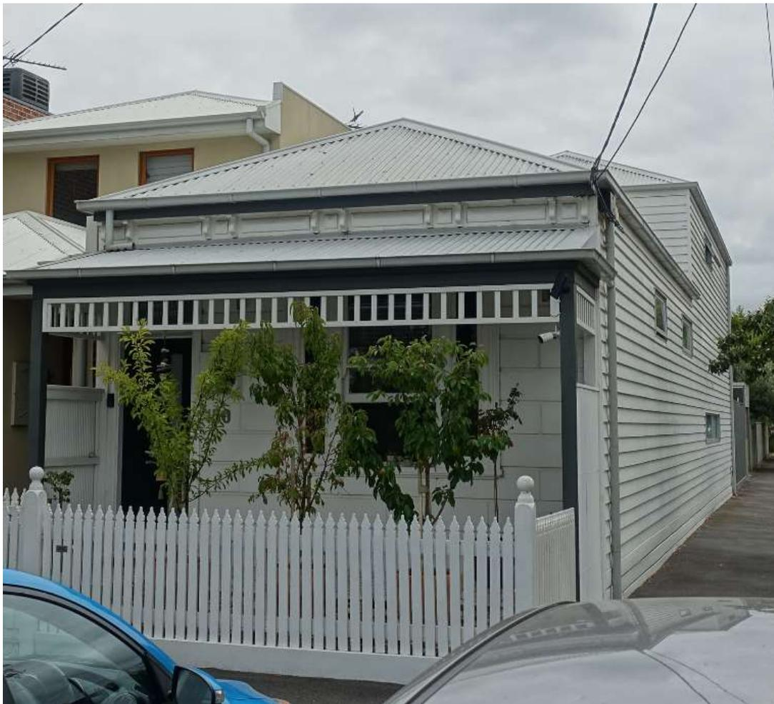
*Figure 8. Significant house at 150 Farrell Street. Note rebuilt verandah with simplified detail, new front fence and two-storey rear addition.*
