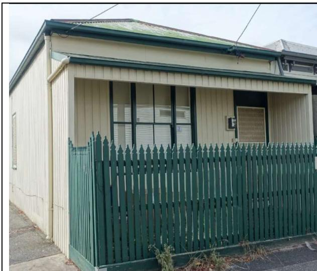
*Figure 47. 12 Derham Street. Alterations: removal of chimneys, verandah, eaves brackets and front window; recladding in vertical boards.*
