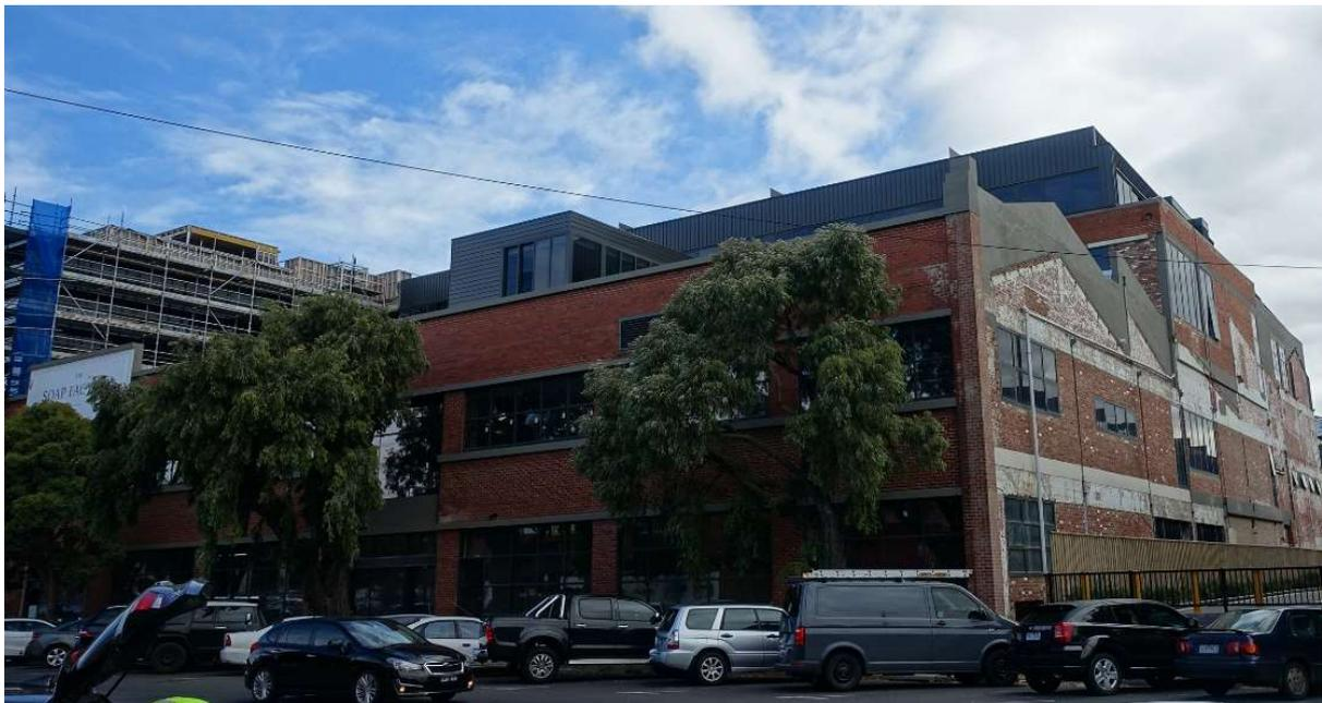
Figure 25. 14 Woodruff Street, following demolition of its southern neighbours. The profiles of the gabled and sawtooth roofs of the adjacent building(s) are visible on the south wall.
