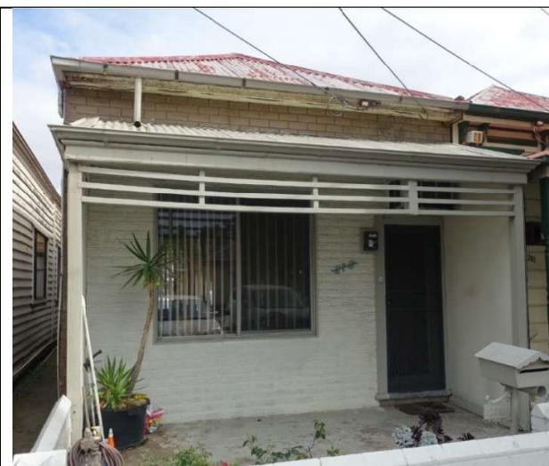
Figure 51. 279 Ross Street. Alterations: removal of chimneys, eaves brackets, verandah posts and ornament, reformatting front window, recladding in fake brick.
