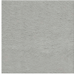
F02 GRAY RENDERED WALLS External brick walls on east elevation covered with gray render (darker shade than F01)
