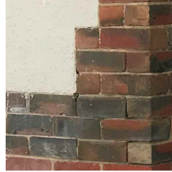
F04 EXISTING RED BRICK Ornamental entry door contour and half height section below windows on east elevation
