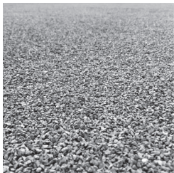
F18 BALLAST ROOF Ballast roof finish to the roof of the southern pavilion.
