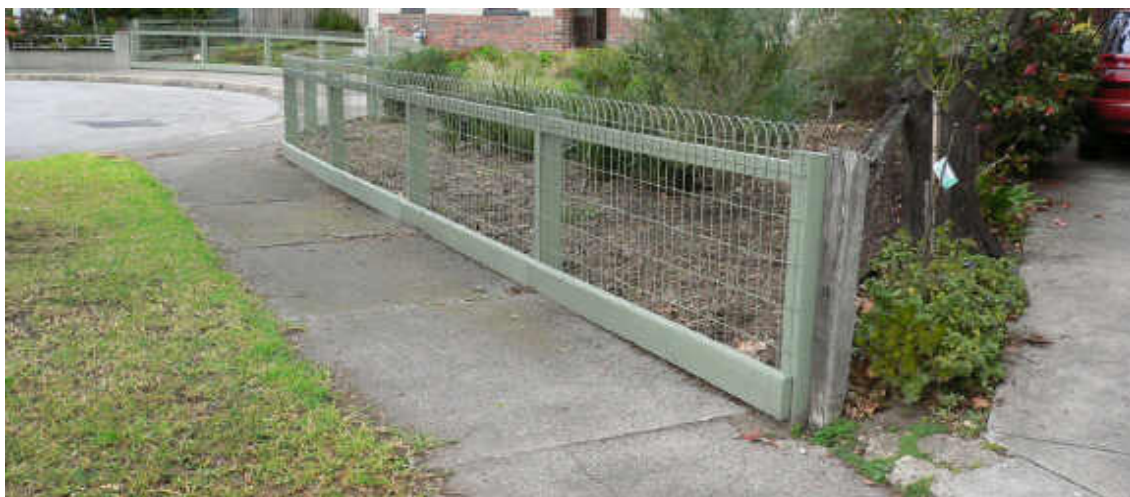
Figure 18: New woven wire fence on timber framing set to a low height (acceptable)
