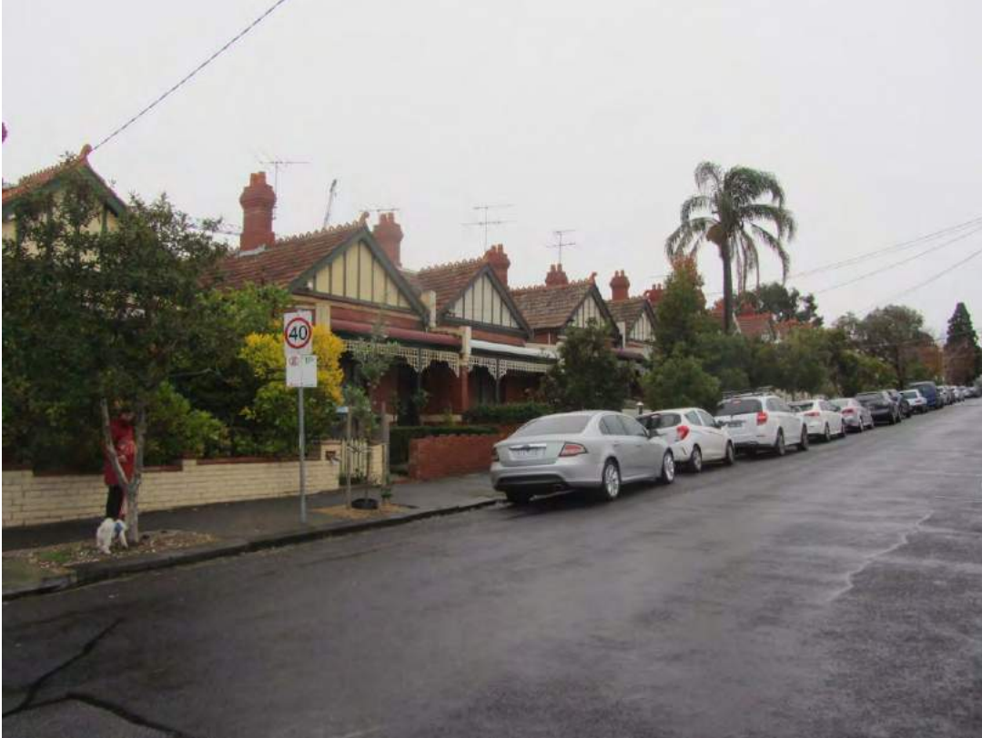
Figure 11. Houses at 10-36 Lambeth Place. Note the high degree of intactness and similarity of design and detailing. This detailing is more typical of the period when compared to that of Barkly and Blanche streets group.
