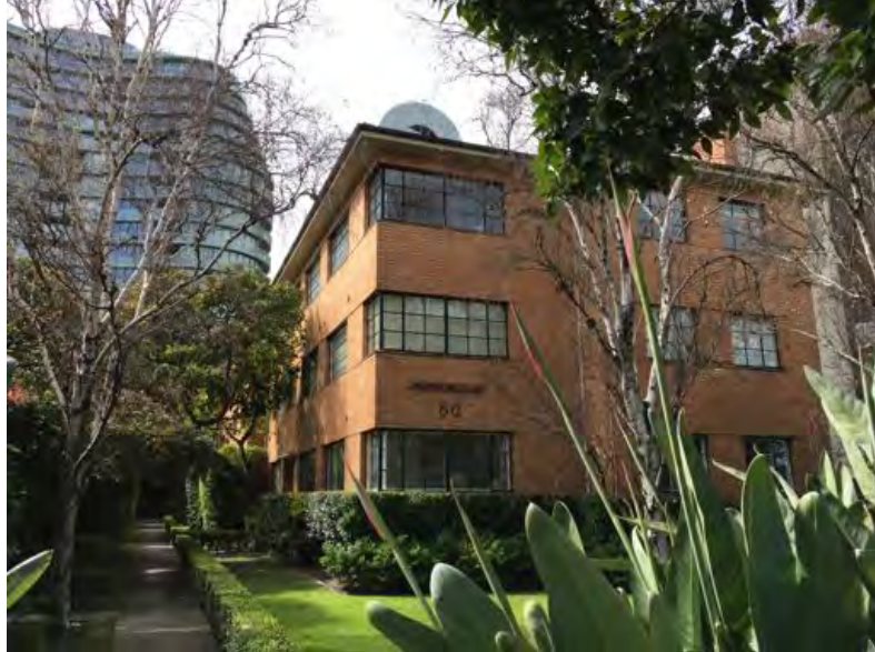
Kinfauns, 60 Queens Road, which is situated at the south of the site.
