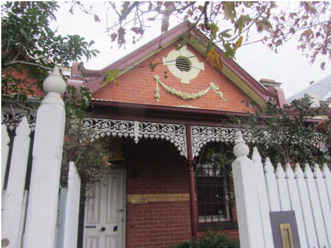
Figure 2. Showing decorative detailing common to 110-112 Barkly Street and 2-6 Blanche Street (oculi and swagged garlands on gable end, verandah posts and cast iron frieze, cream brick banding).
