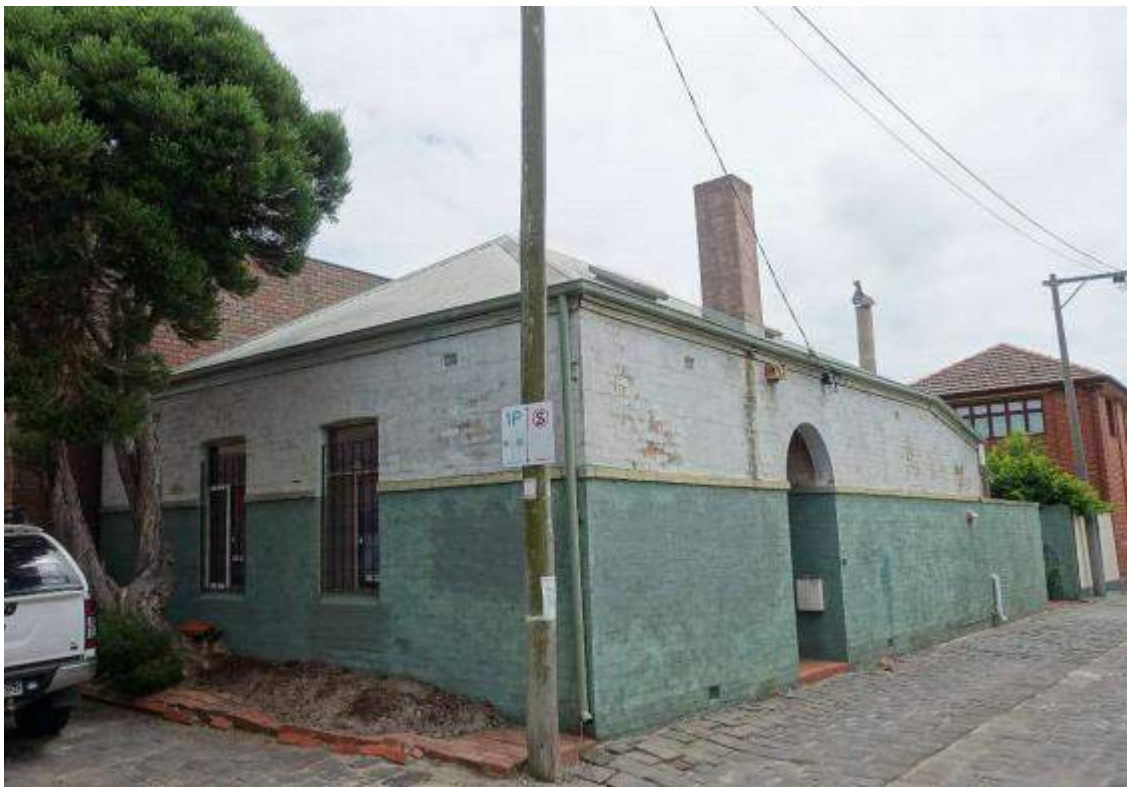
Figure 1 Streetscape photograph of 207 Little Page Street, Middle Park (Source: Ms Schmeder's expert report, page 18)
