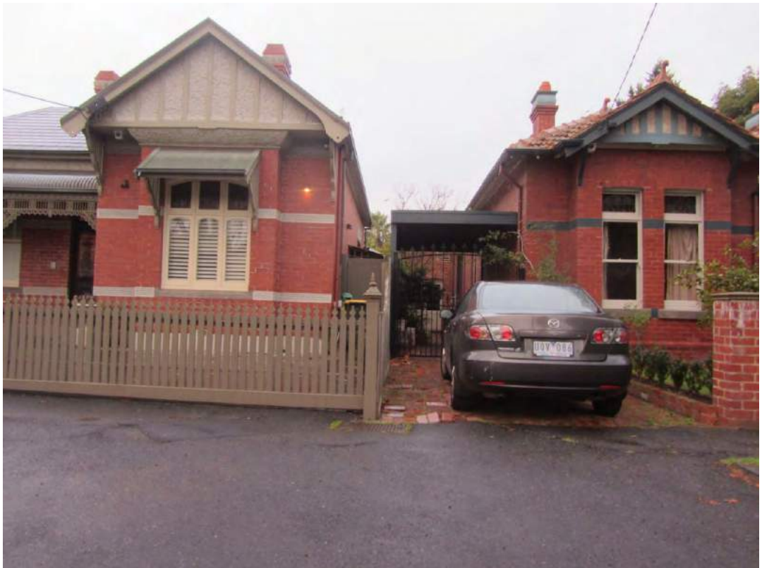
Figure 10. Houses in the row at 1-15 Charlotte Place, St Kilda, constructed c.1905-1907 in the St Kilda East Precinct (HO5).
