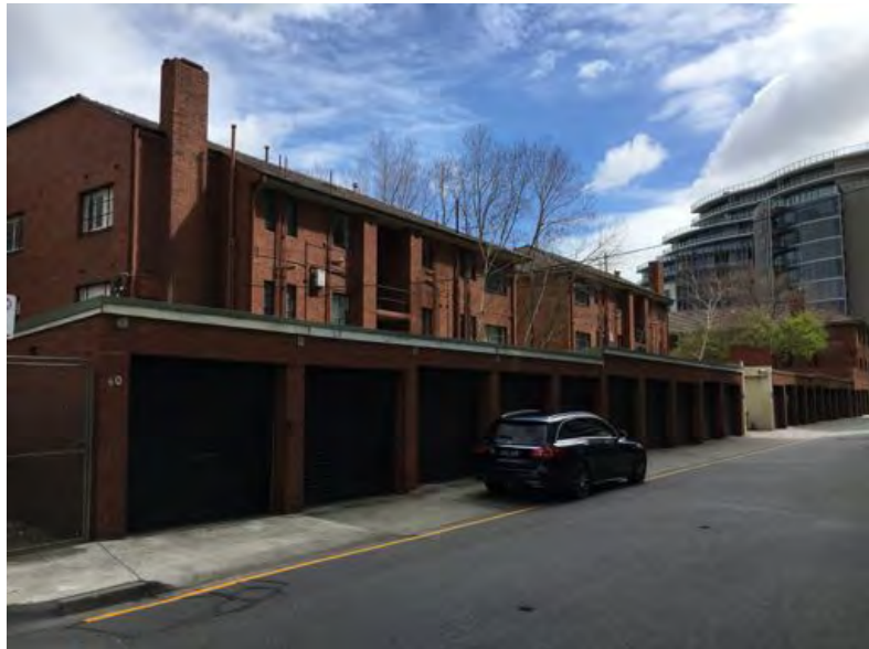
The rear of Kinfauns and Kinross, viewed from Queens Lane. Visible in the foreground are the 23 single-car brick garages of the complex. The rear of Glen Eagles is partially visible at right.
