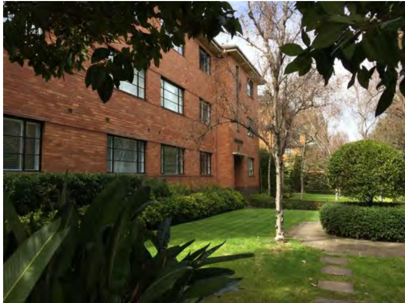
Glen Eagles, 58 Queens Road, west elevation facing Queens Road. The other two blocks in this complex, Kinross and Kinfauns, are partially visible at right.
