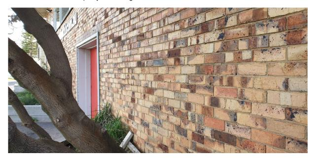
**Figure 9.** Photograph showing cream clinker bricks laid in stretcher bond taken from the south west corner facing Port Phillip Bay in 2020 (Source: Context)
