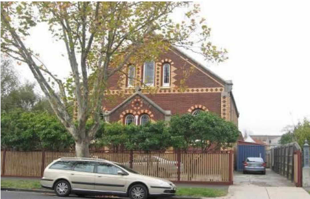
Figure 4 Baptist Church at 16 Crimea Street, St Kilda (1876) Individual Significance (Citation No.86) within HO6 St Kilda East precinct
