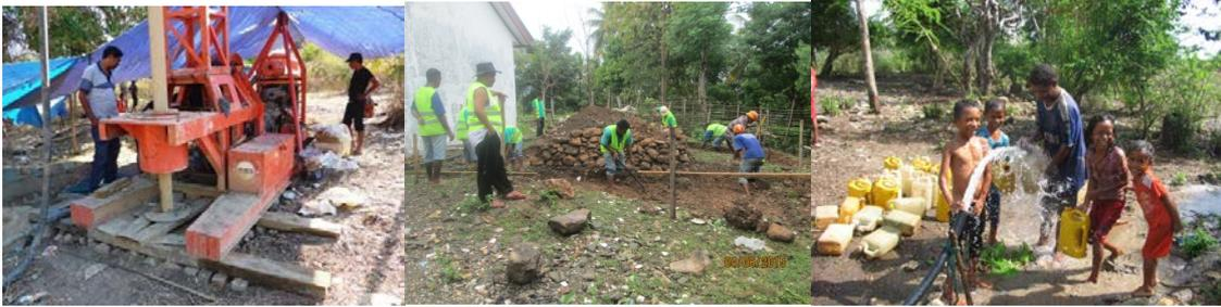
**Drilling the bore, foundations for the elevated tank and the first water from the bore**
