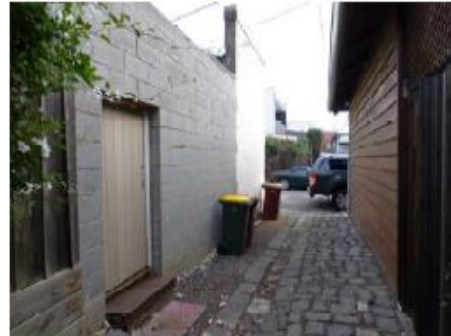
Looking along the Road towards Coventry Place
