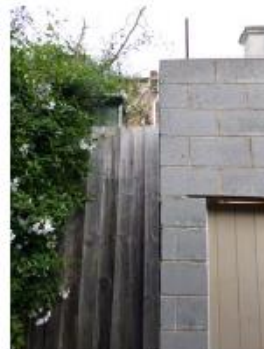
Looking along the boundary between 378 & 380 Coventry Street
