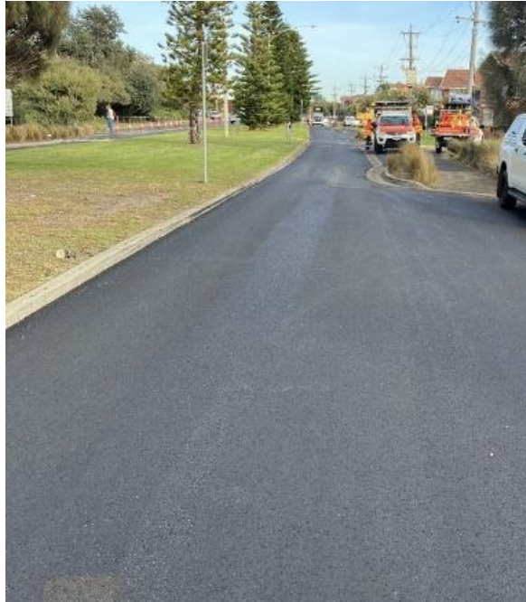
Example of road surface upgrade
