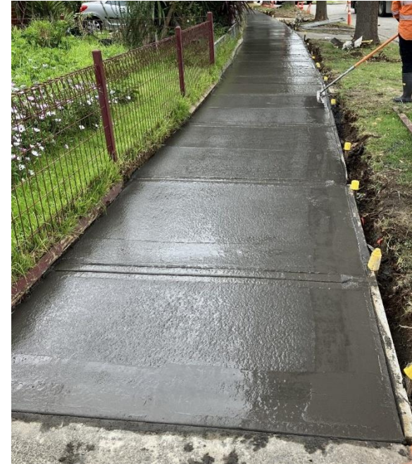
Example of footpath renewal
