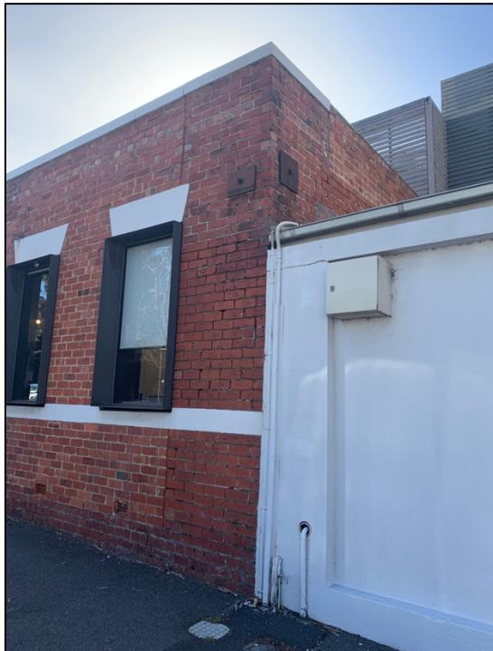
Figure 13 The southern brick extension (without parapet detailing) with the roof addition partially visible. Note the areas of brick that have been reworked, with expansion joints introduced to the brick face that separate different generations of pointing to brickwork.
