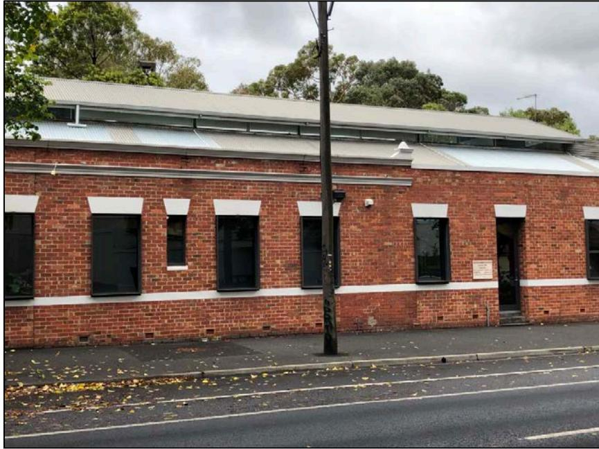
*Figure 10 The Ferrars Street elevation of the subject building. The metal window shrouds and glazed windows are non-original. The two cornices that span the parapet of part of this elevation are of a modern segmented construction, suggesting they date from the same period as the window shrouds, ie they are not of traditional construction. The roof has been extended to form a first floor. The brick facade has been subject to extensive change.*
