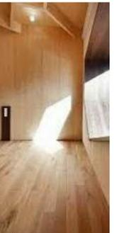
CLT soffit and internal skin
