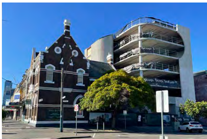
Image 11. Former ANZ Bank building with a new commercial development under construction at the corner of Clarendon Street and Bank Street.
