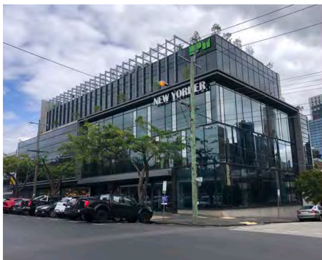
Image 40. Contemporary multi-storey commercial development on Clarke Street.
