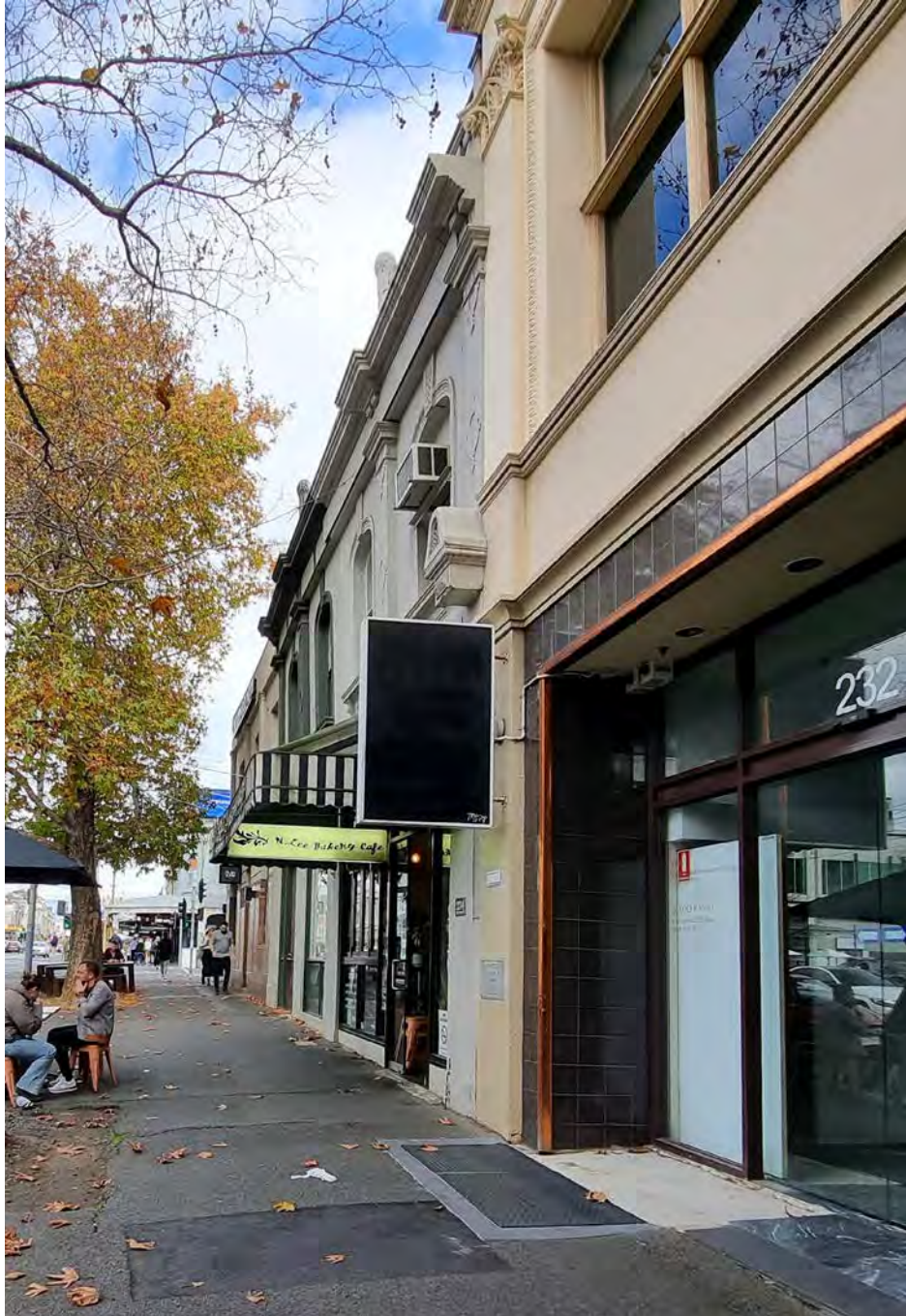
Image 27. View of heritage shop residences along Clarendon Street.
