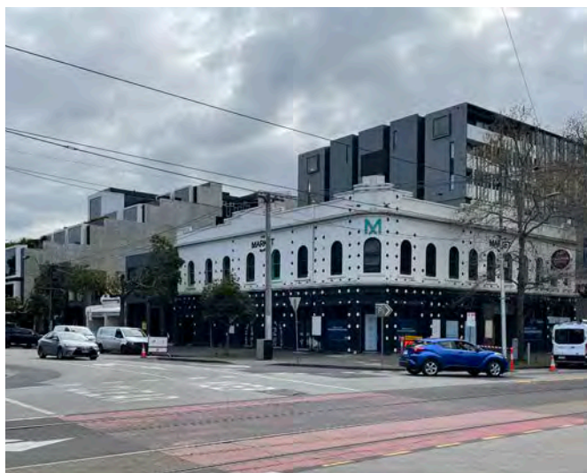
Image 46. Hotel South Melbourne at the corner of Clarendon Street and Market Street with contemporary development in the background.
