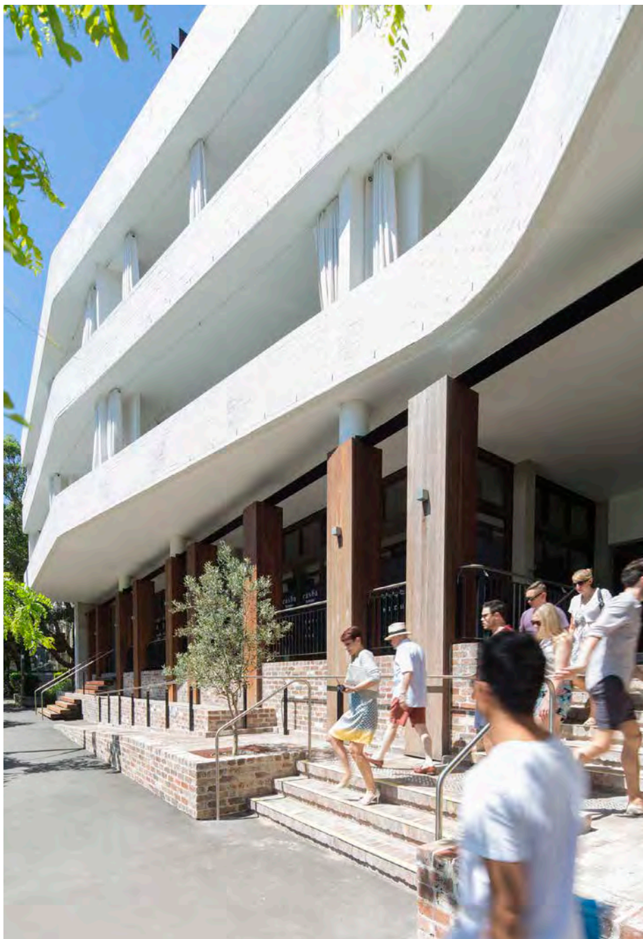
Image 26. Entrance to Casba in Waterloo, Sydney. A successful transition area is achieved by integrating ramps and stairs with the overall façade design and the use of high quality natural materials. The curve in the facade creates a cue for direct people to the entrance and enables increased light penetration.
