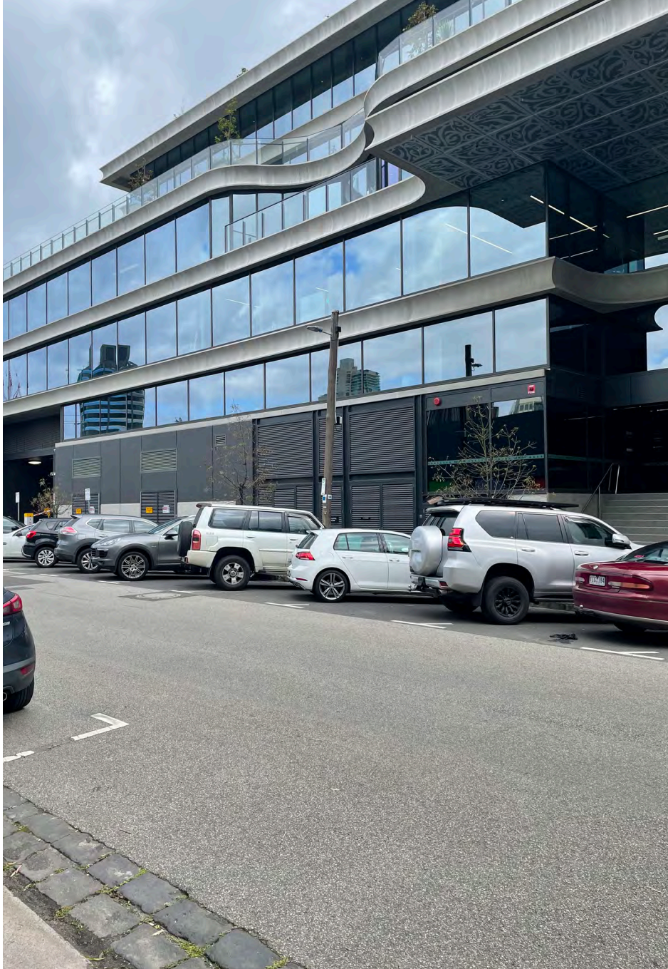
Image 20. The design response to raised floor levels in combination with inactive frontages results in a poor quality outcome for the public realm and equitable access.
