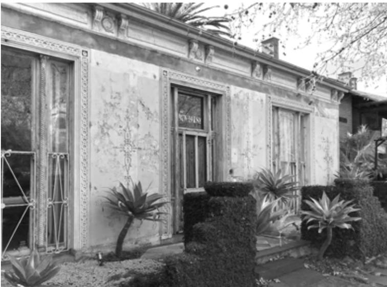
*Photo 2. The removal of a c.1950s addition at the front of this house in Blessington Street, St Kilda revealed the original intact Victorian era façade. Outlines of the removed verandah and walls and some of the colour schemes, as well as the lower sections of the walls (now covered in vines) were left as evidence of this change.*
