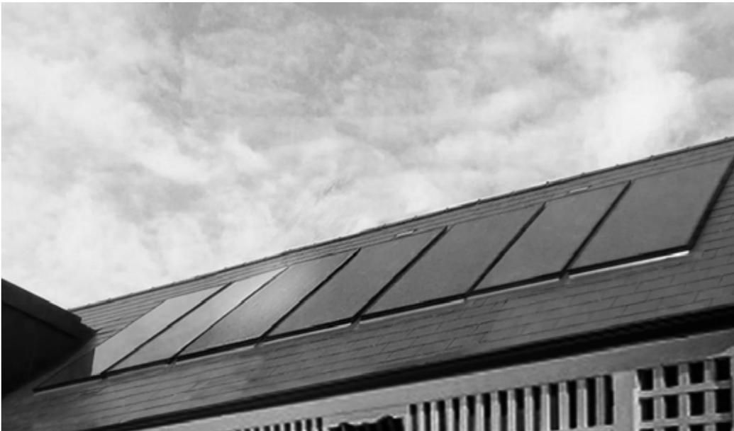
*Photo 22. An example of frameless solar panels on a slate roofed building*
