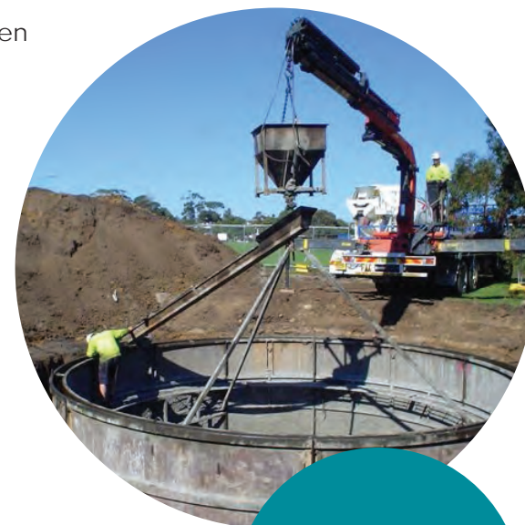
Installation of below-ground tank in Elwood Park 2012
