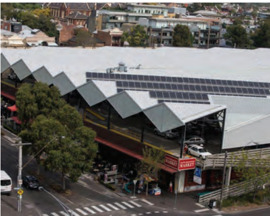
The 34kW solar PV array at South Melbourne Market (Source: City of Port Phillip).
