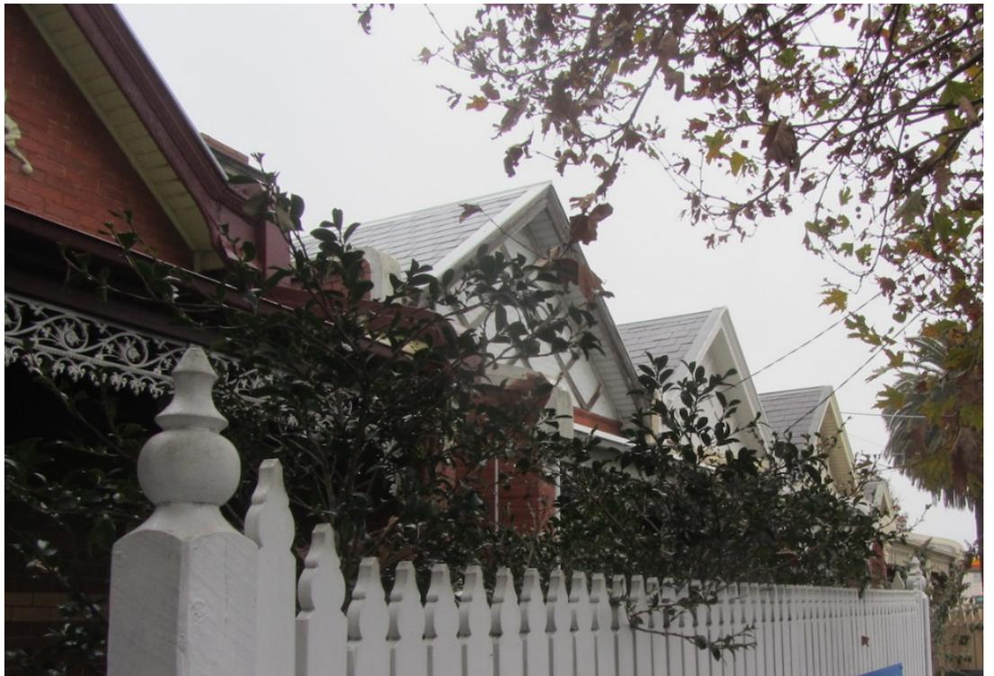
*Figure 6. 114-118 Barkly Street, showing slate roofs to all, and alternate gable end decoration on 114-116 Barkly Street.*
