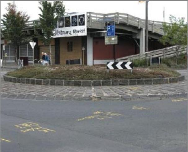
**Photo 31.** *Roundabout in Cecil Street, South Melbourne which uses recycled bluestone pavers*
