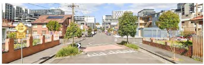
An example of a chicane in Richmond on a typical width street (approximately 15m) that creates space for two trees, understorey planting, and the continuation of two directions of vehicle traffic (Image Credit Google Street View).
