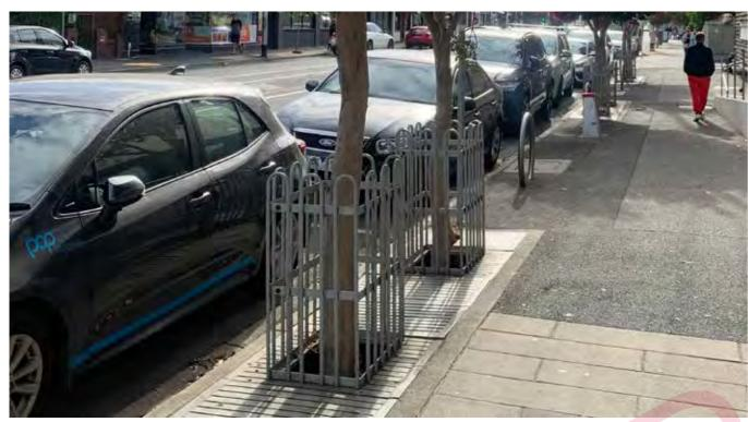
An example of tree cut outs on Carlisle Street with trees planted into pits large enough for connected soil between pairings.
