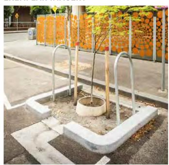
This example shows how a spoon drain between driving lanes and parking bays can direct stormwater to the outstand (Image Credit City of Melbourne)
