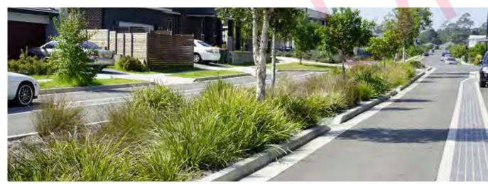
A vegetated swale in a central median strip in Bungarribee, including breaks in the kerb for passive irrigation (Image Credit Blacktown City Council)
