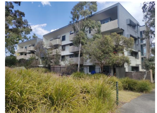
An apartment block in Port Phillip.
