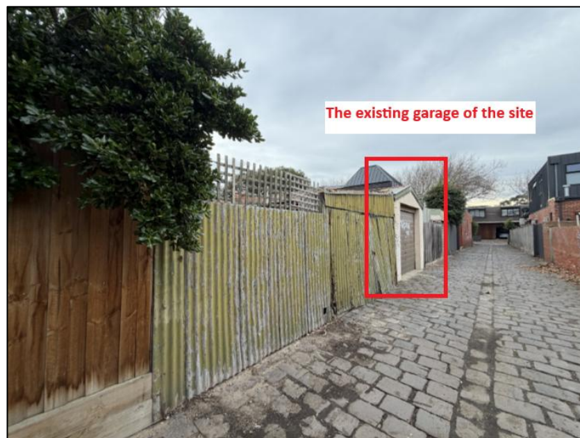
Figure 15. View of the rear laneway, facing towards Lawson Street, showing the site's rear garage (Source: Council, dated 16 June 2026)
