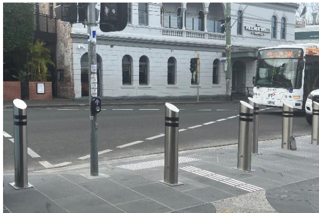
New safety bollards installed on Acland Street
