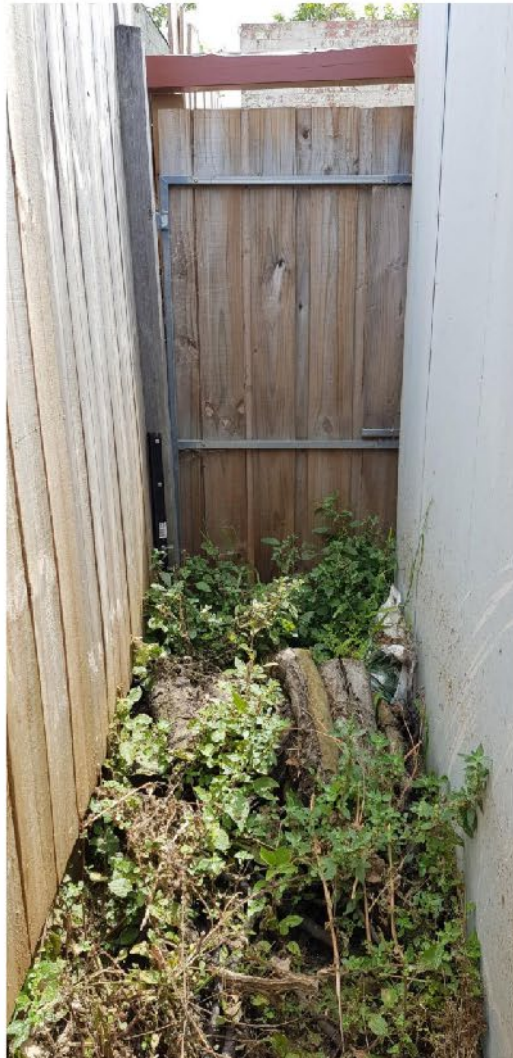
Showing the disused gate at the southern boundary of 48 Nimmo Street
