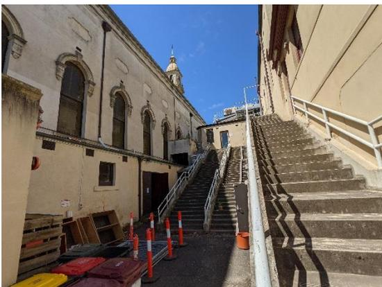
Figure 71 Former service yard with retrofitted concrete fire stairs
