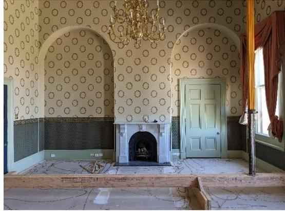
Figure 37 Mayor's Room, as remodelled to a Victorian style in 1991, with temporary structural propping installed and carpet removed
