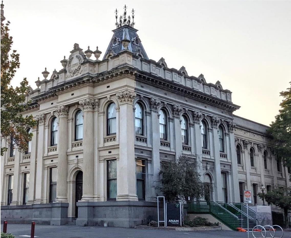
Figure 23 South-east corner of block (former post office) showing step down to the former council rates office (1938, right), and distinction between ochre skim coat (left) reintroduced in 2000s conservation programme and bare (grey) pressed cement render (centre)
