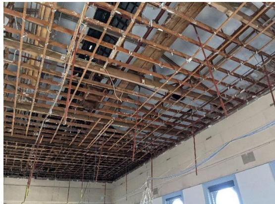
Figure 51 Lodge Room ceiling joists with remnants of earlier raked ceiling behind
