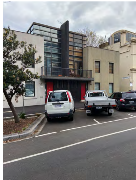
229 Rouse Street - 3 storey building directly next to subject site
