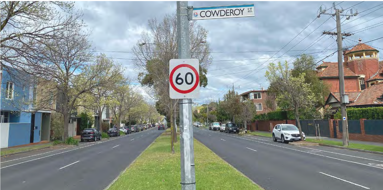
Figure 27: Canterbury Road in Middle Park is a Moderate Movement Corridor.
