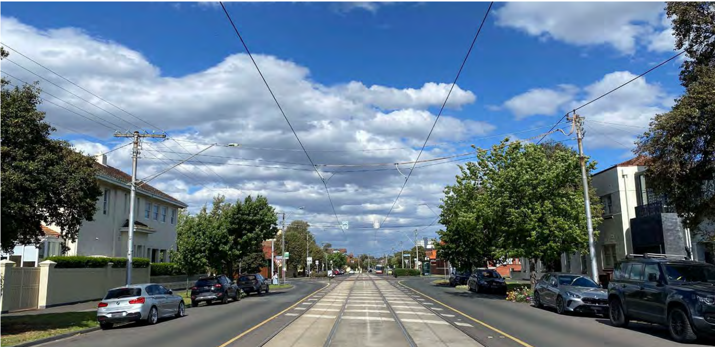
Figure 30: East of Mills Street, Danks Street in Albert Park is an example of a Movement Street
