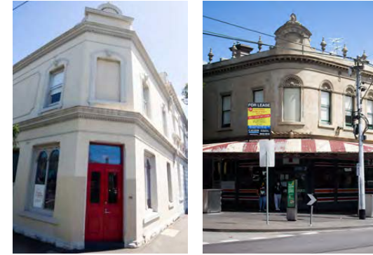
Figure 9: Buildings in South Melbourne with splayed corners and dual frontages addressing two streets and creating a landmark.
