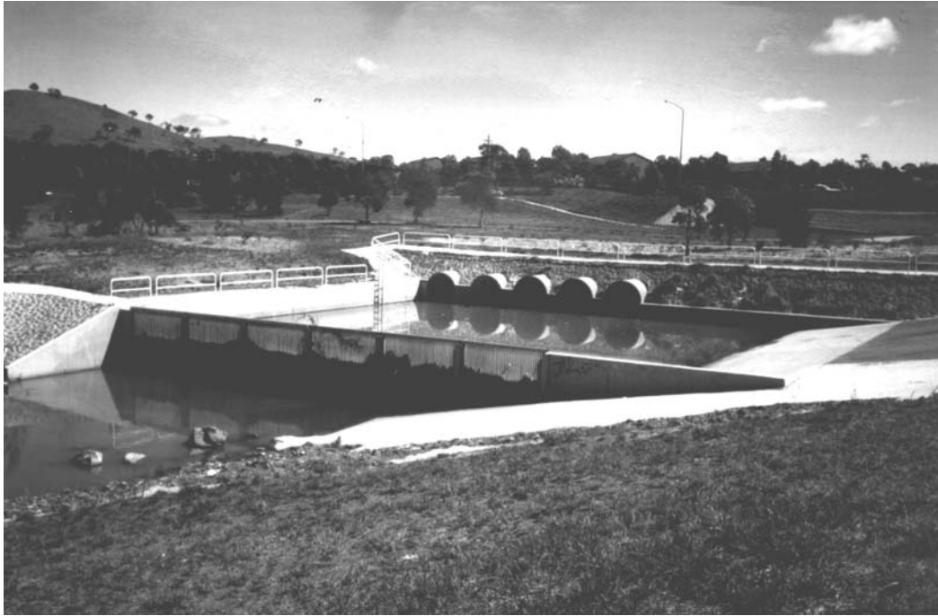
Figure 7.13 Gross pollutant trap, Tuggeranong Lake, Canberra.
