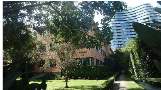
Kinross (no. 59), Queens Road façade from entry path. Despite modifications to the original courtyard, the landscaped setting and path configuration remain intact.
