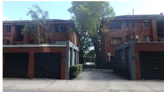
Queens Lane façade showing vehicular entry between Kinross (no. 59) and Kinfauns (no. 60). The additional garages along the Queens Lane boundary had been constructed by 1945.
