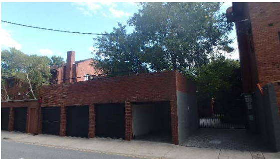
Queens Lane (rear) façade showing Glen Eagles (no. 58) to the right and original single car garages (x4) to the left.
