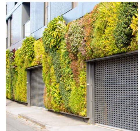
Green infrastructure - roofs, walls, WSUD
