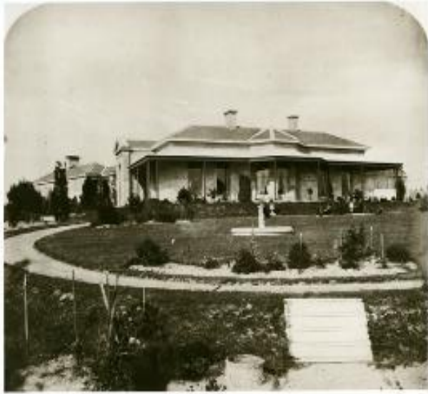
Westphalia Villa 1872 182-190 Alma Road, St Kilda East Donald McDonald (Photographer) Port Phillip City Collection sk0441
