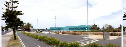
400 boat double width dry storage: 3 level at 12m high and 200m long
