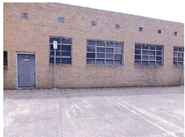
The southern wall of the building at 34 Tope Street
