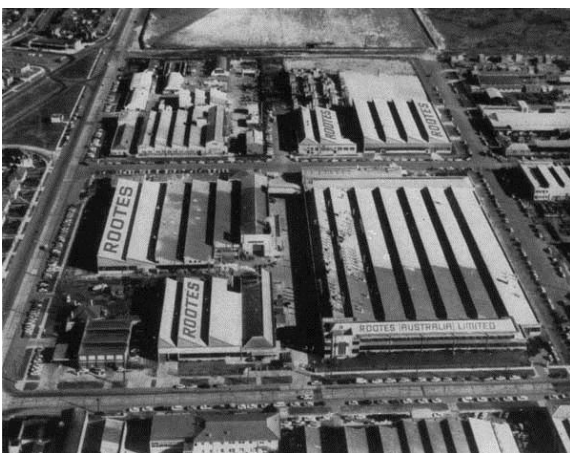
Figure 2 – Rootes factory in 1950s looking west, showing recent extensions with light roofs (Source: The Supreme Sunbeam)
