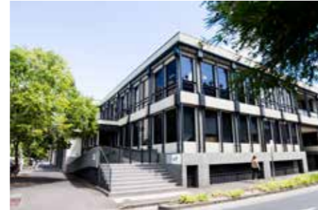
Late 20th century office building
