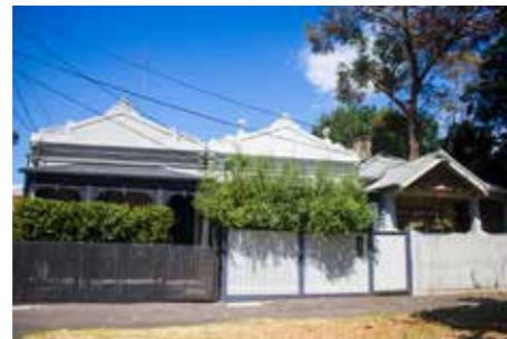
Victorian worker's cottages
