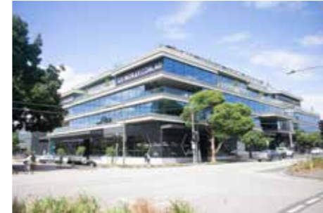
Large format commercial building
