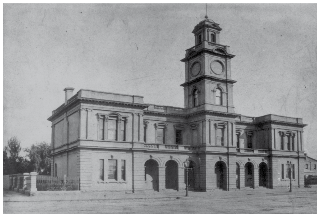
View of Port Melbourne Town Hall with no clock c1886. PPCC pm1601
