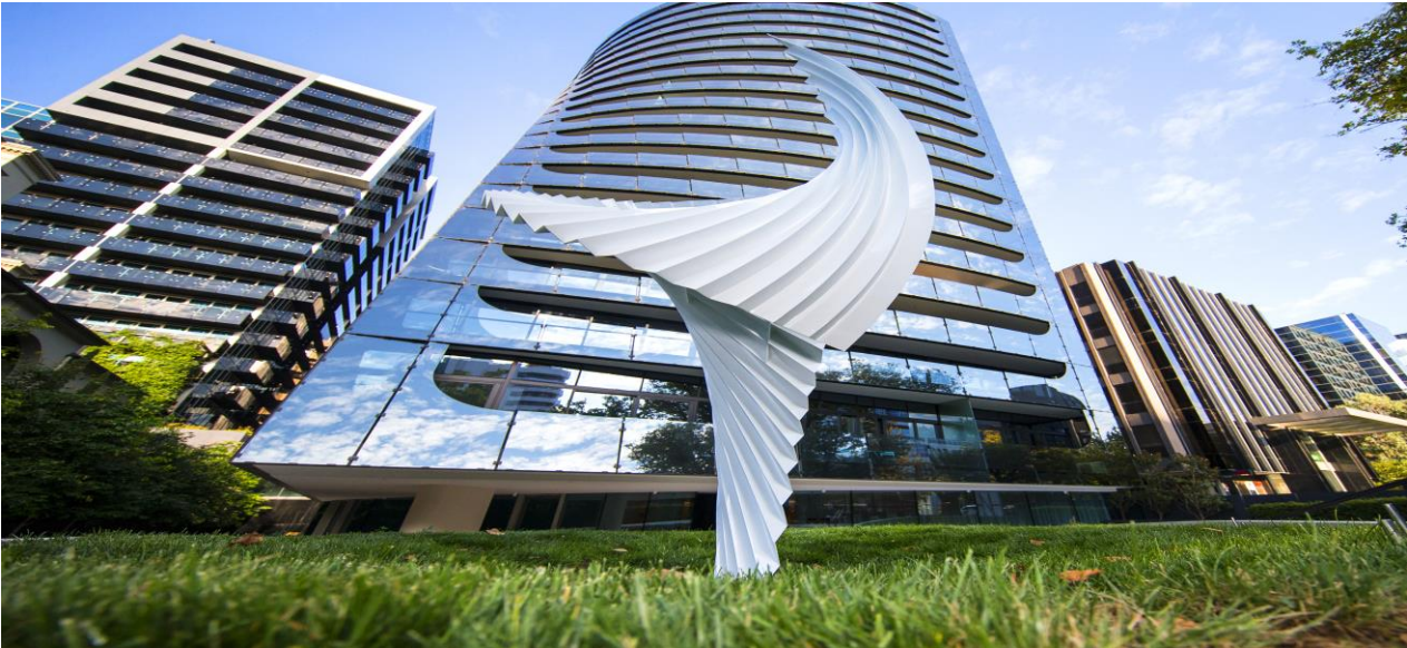
Matthew Harding Opera 2019 450 St Kilda Road, Melbourne. Photo courtesy ADA Consulting
